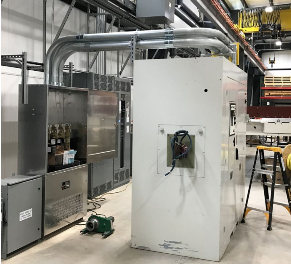
Figure 48. Picture of the 1MW 1 to 3 KHz induction power supply during installation adjacent to the large scale restraint.
