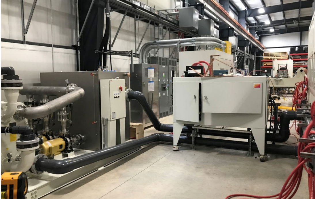
Figure 51. Picture of 1MW power supply connected to the tool along with the water supply with pump connected to the power supply and tool
