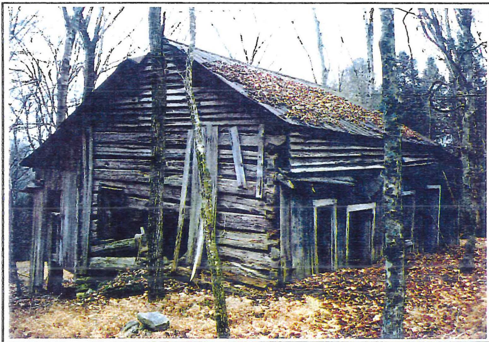
Plate 42: 61A - View looking southeast at log-and-frame construction.
