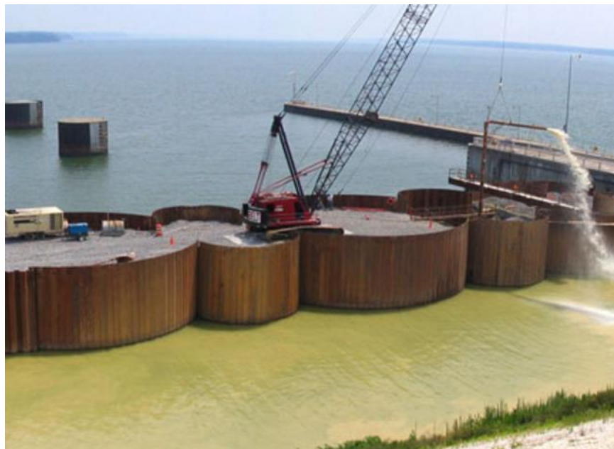
Figure 8. Construction of the Kentucky cellular cofferdam (C. J. Mahan Co., 2017).
