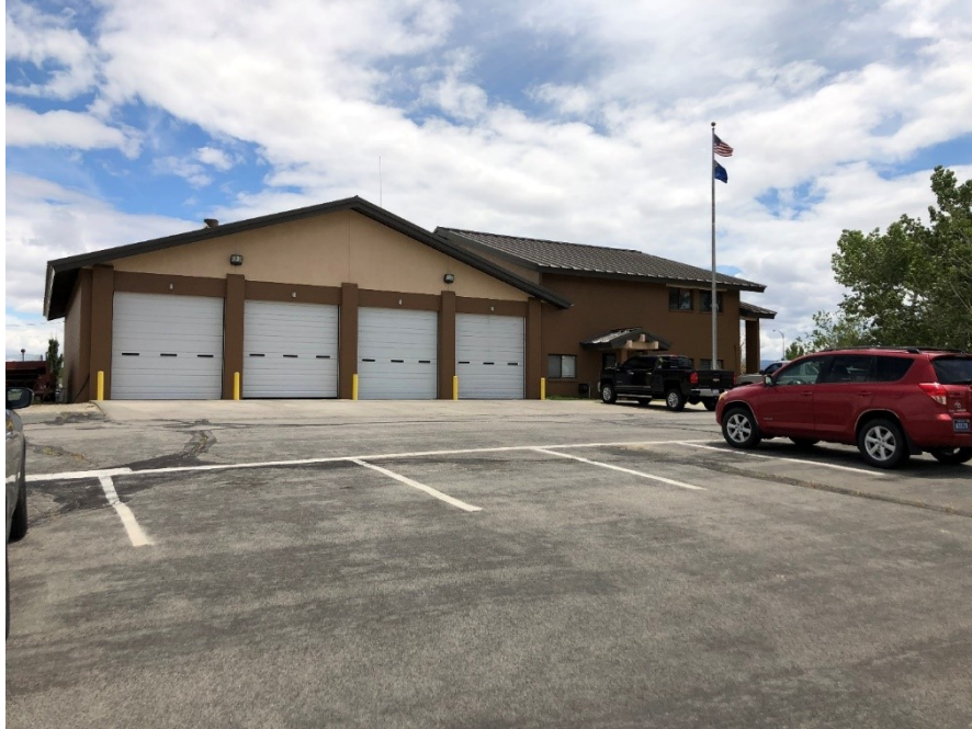
Figure 31 - Hawthorne Fire Department Station.
