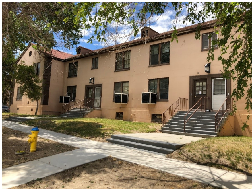
Figure 34 - Admin General Purpose Building at Hawthorne Army Depot.
