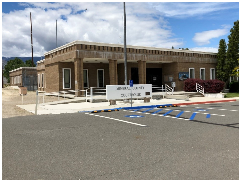
Figure 28 - Mineral County Courthouse/Sheriff's Office Complex.
