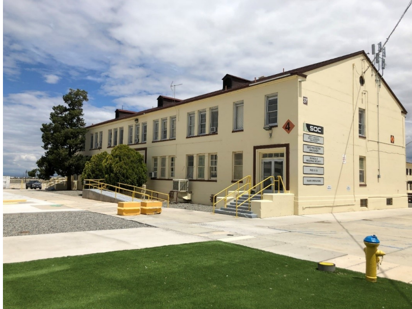
Figure 35 - SOC Admin General Purpose Building at Hawthorne Army Depot.
