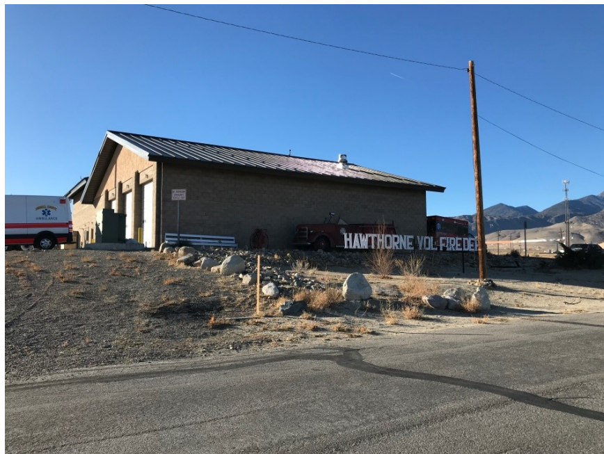
Figure 30 - Hawthorne Fire Department Station.
