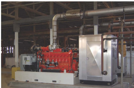
Ammonia/water absorption chiller integrated with a CHP system consisting of two reciprocating engines. Photo courtesy of Energy Concepts.
