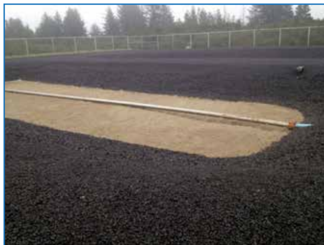
Figure 2.1 Camp Rilea Rapid Infiltration Basin
