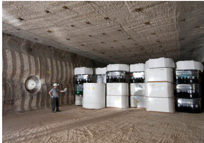
Fig. 4.1. Disposal operations for Transuranic (TRU) waste at the Waste Isolation Pilot Plant (WIPP). (Reproduced from Hansen and Leigh [2011] .)
