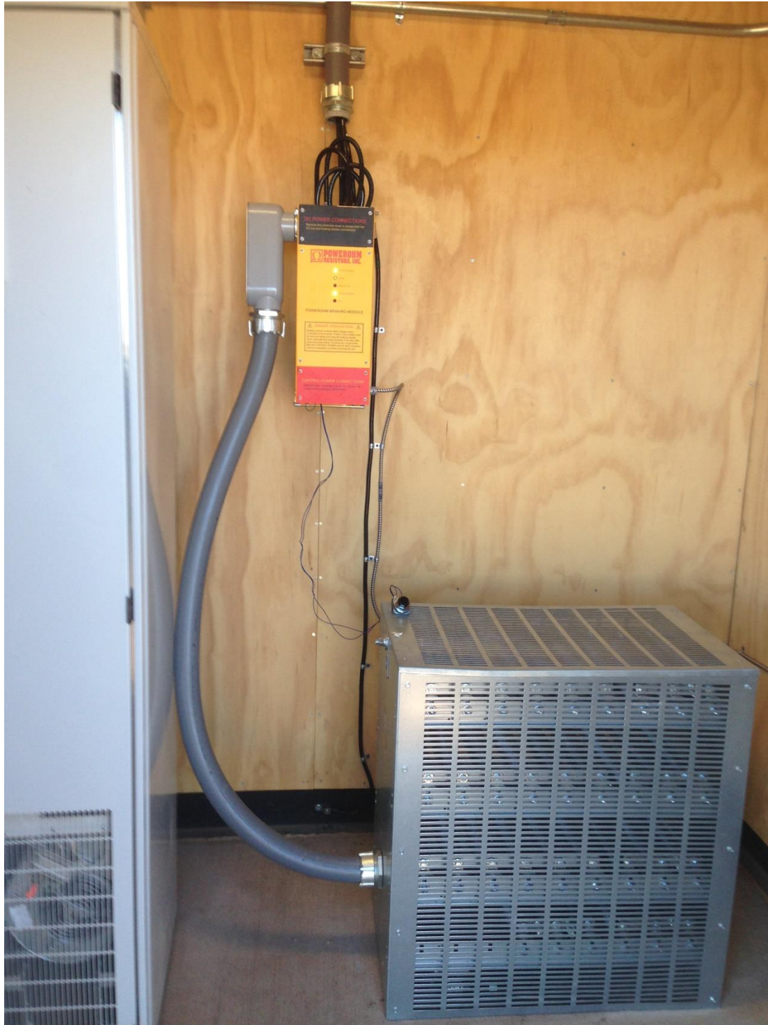
Wired Brake chopper and resistor bank.
