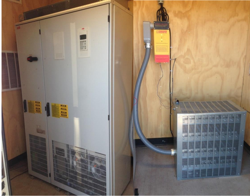
Figure 13. Variable Frequency Drive and Brake Chopper
