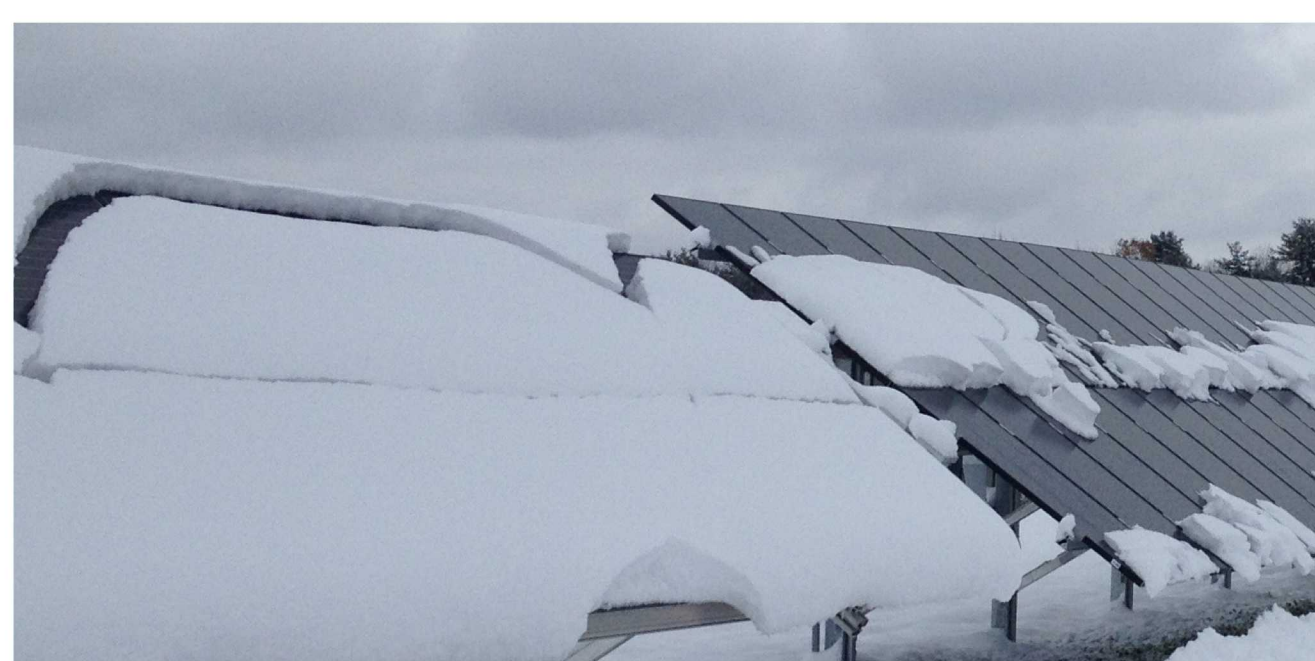
Figure 5. Differential snow shedding across modules creates mechanical stress
