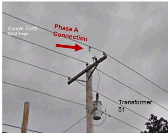
Figure 14. Phase A connection for transformer 51
