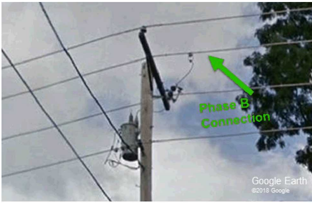
Figure 13. Phase B interconnection of transformer 53
