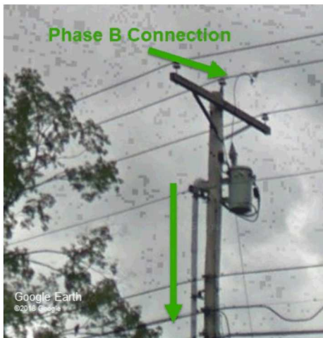
Figure 9. Transformer 80 from Figure 8 verified in Google Street View to be connected to Phase B as predicted by spectral clustering.
