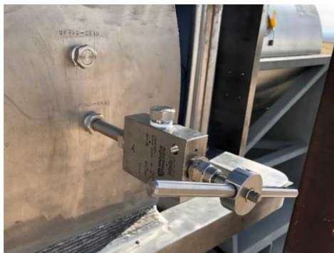
Figure 14: Large three-way sample valve installed on the drain port.
