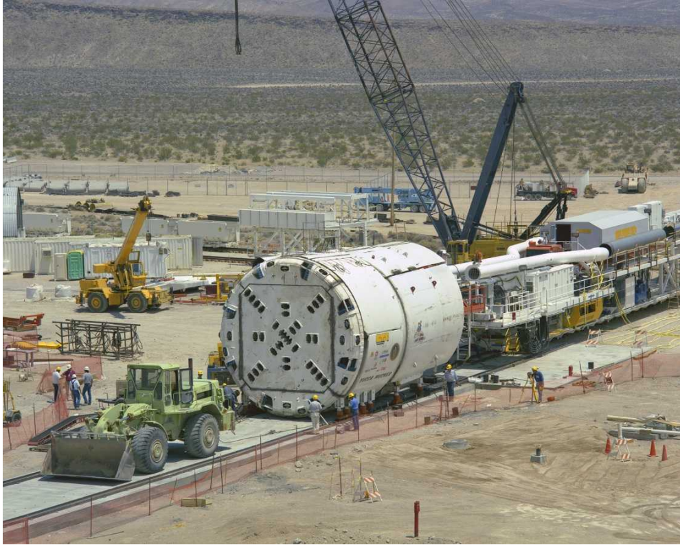
Figure 2-1. Open-type double-shield TBM with trailing gear, during assembly, Yucca Mountain, Nevada (diameter 7.6 m)
