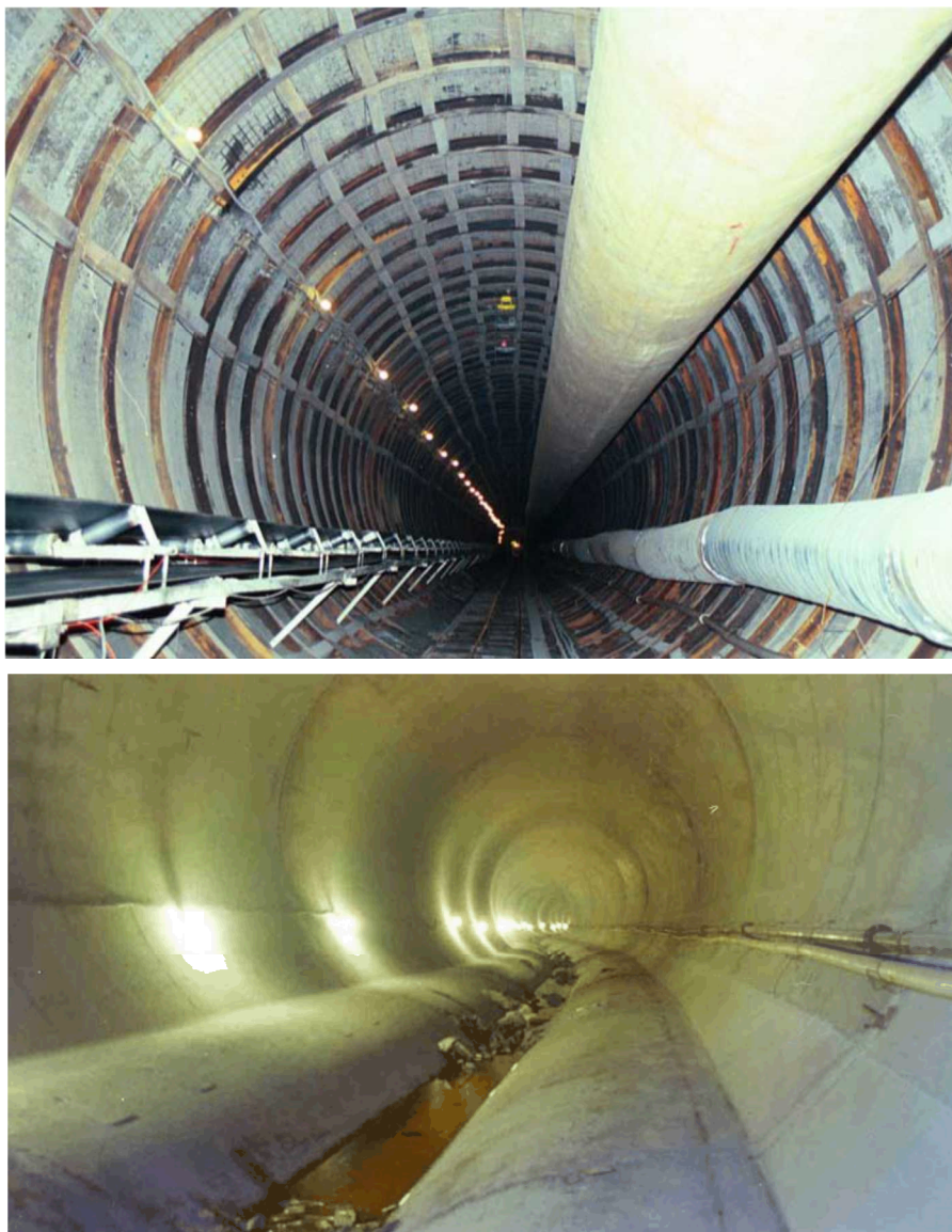
Figure 2-6. Mill Creek Tunnel Phase 2 showing steel ribs and lagging support (upper) and final cast-in-place concrete liner (lower) (with permission, HMM 2010)
