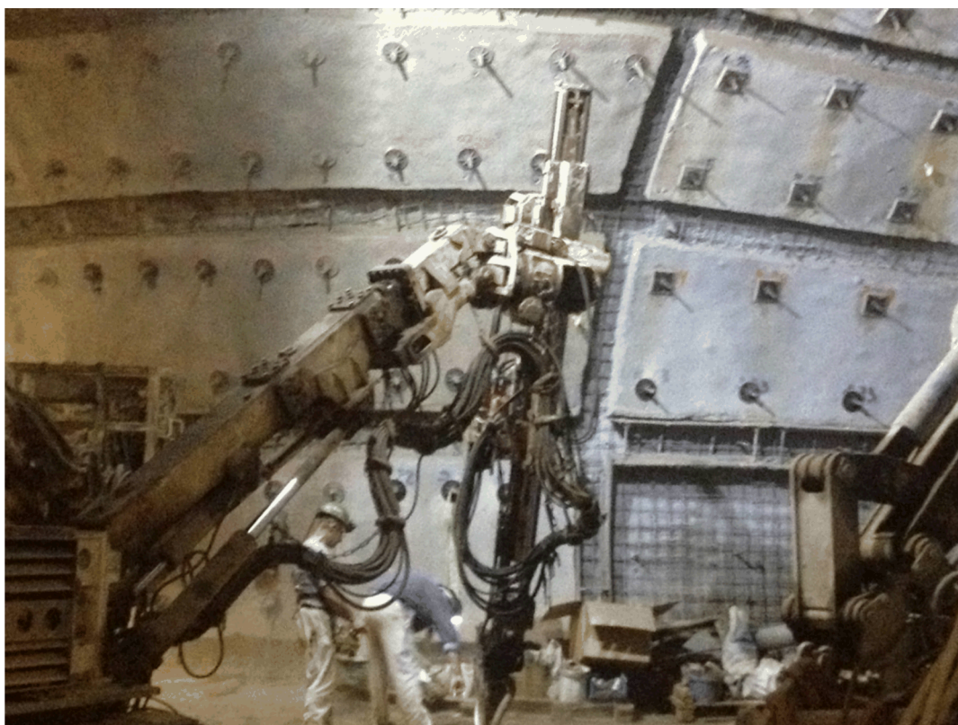
Figure 2-5. Yielding initial support (wire fabric, shotcrete and long rock bolts) just after installation in the Lower Cretaceous clay at the Konrad repository site (depth ~1,000 m)
