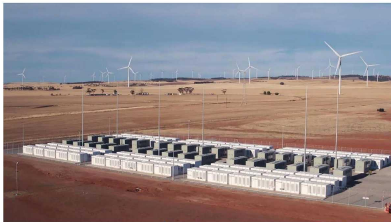
Tesla 100 MW / 129 MWh ESS Australia - Grid stability
