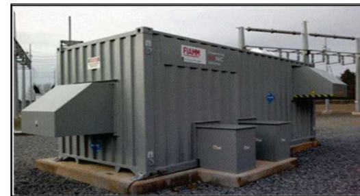
FIAMM 222-kWh System Duke Energy Rankin Substation
