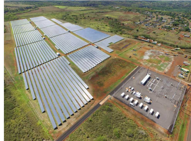
Saft 6 MW / 4.2 MWh ESS Kauai - Grid Stability
