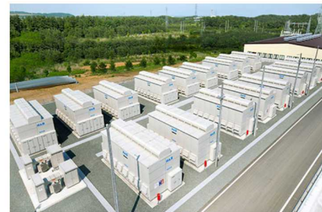
34MW /245 MWh NAS at a wind farm Rokkasho, Aomori, Japan (Source: NGK, 2017)
