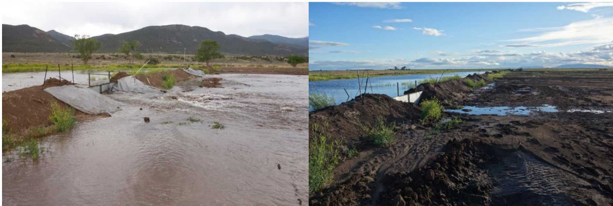
Figure 1-1. Picture of flooding from irrigation system (left) and scouring of the land in front of the gates (Provided by Big Wheel Farm)
