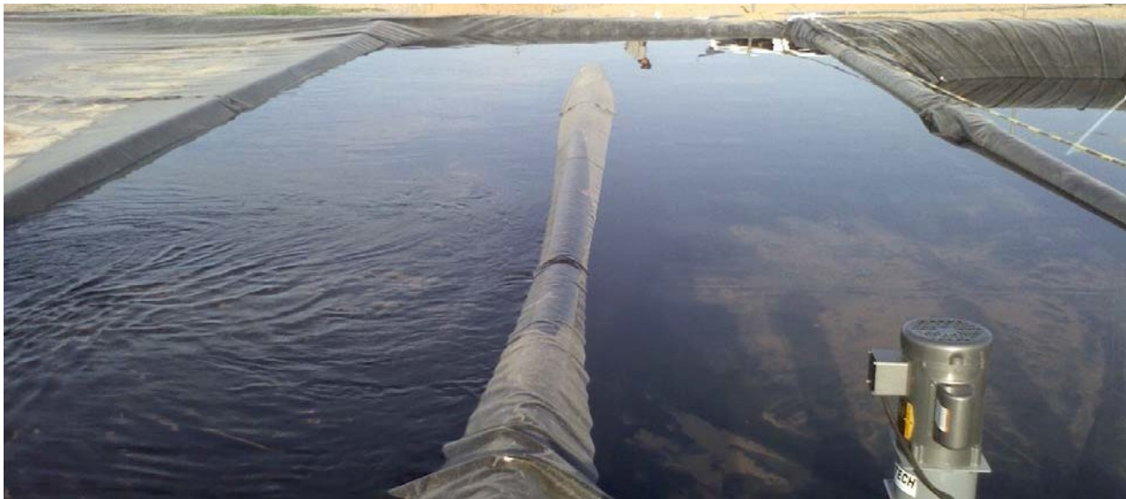
Figure 5. Water directed through basins with air-bag berms.
