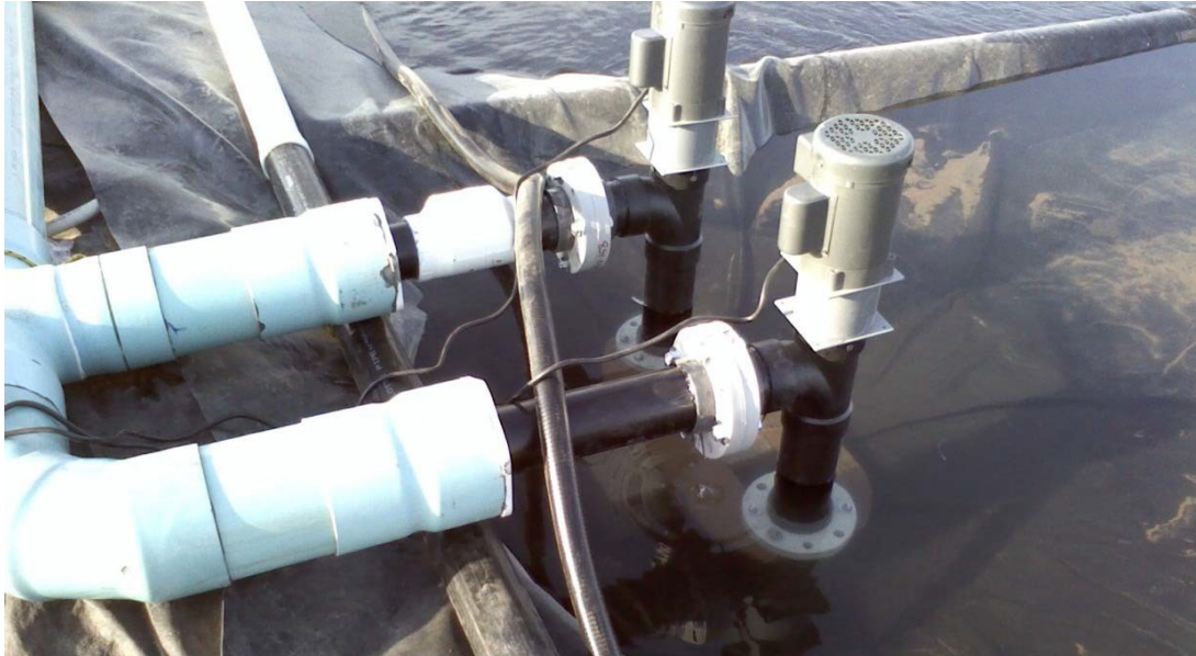
Figure 6. Original propeller pumps for recirculation from the lower channel to the upper channel.
