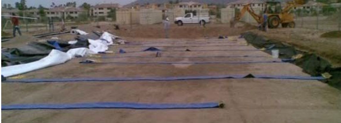
Figure 4. Installation of vinyl lay-flat tubing under liner.
