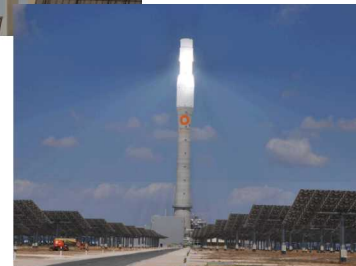
Gemasolar, molten salt, 19 MW e , Spain, 2011
