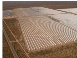
SEGS, 1980's 9 trough plants 354 MW e , CA
