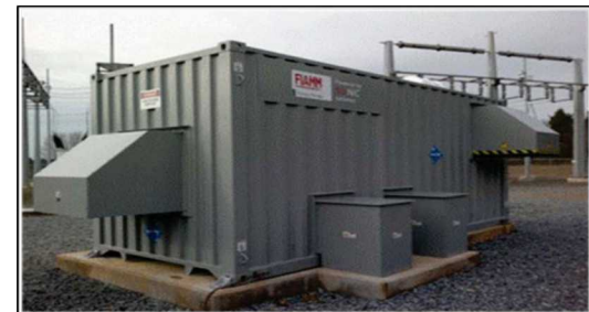
FIAMM 222-kWh System Duke Energy Rankin Substation
