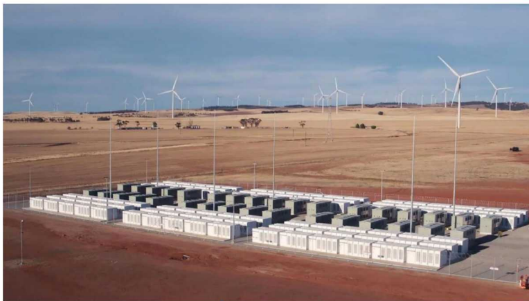
Tesla 100 MW / 129 MWh ESS Australia - Grid stability
