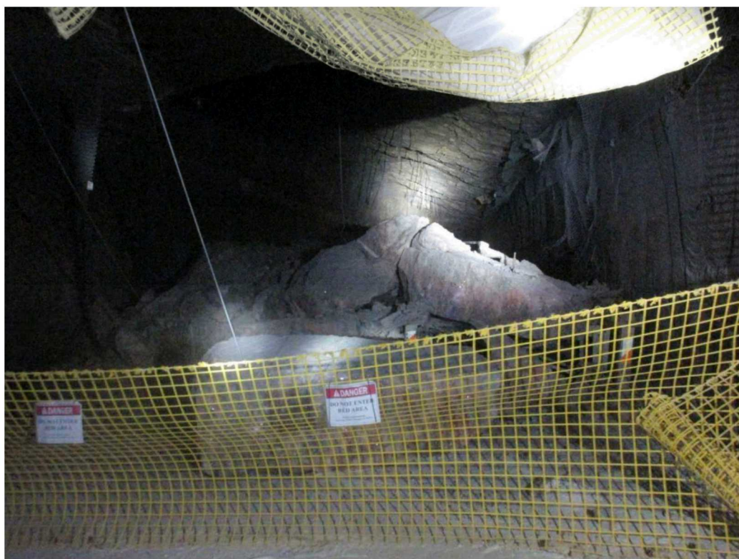
Figure 3. Roof fall in WIPP Panel 7 Room 4 (WIPP Update Nov 4, 2016).
