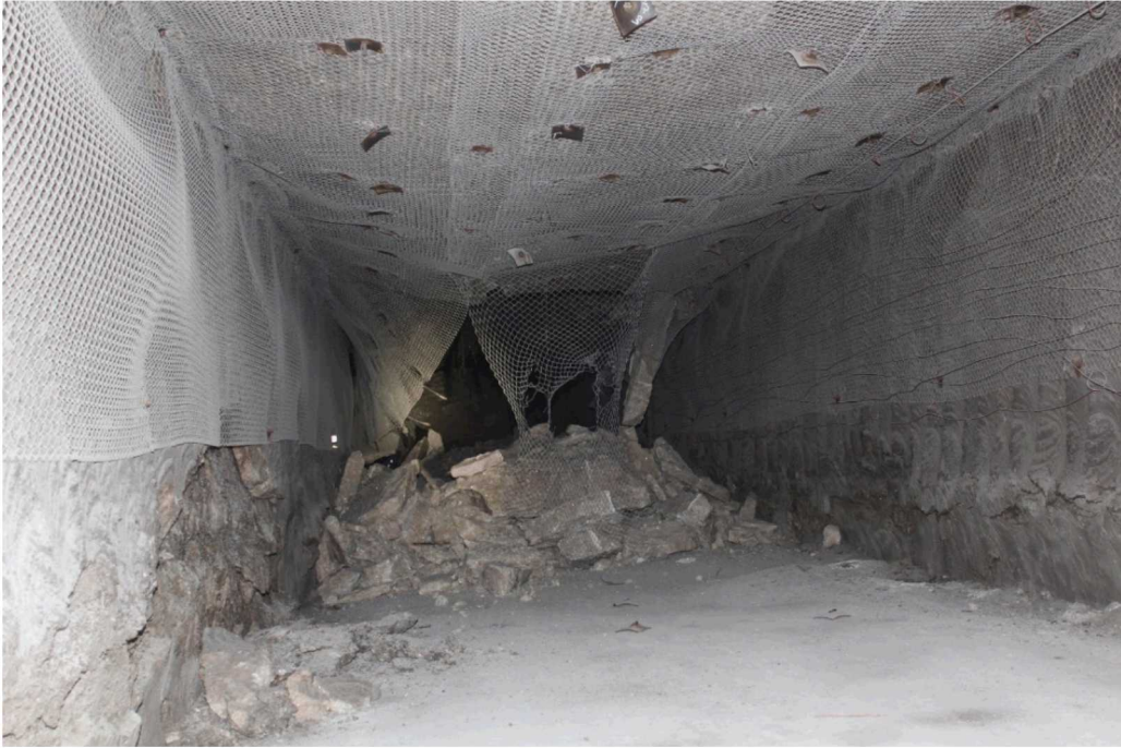
Figure 2. Roof fall in WIPP Panel 3 access drift (WIPP Update Oct 5, 2016).
