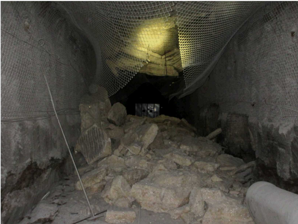
Figure 2. Roof fall in WIPP Panel 3 access drift (WIPP Update Oct 5, 2016).
