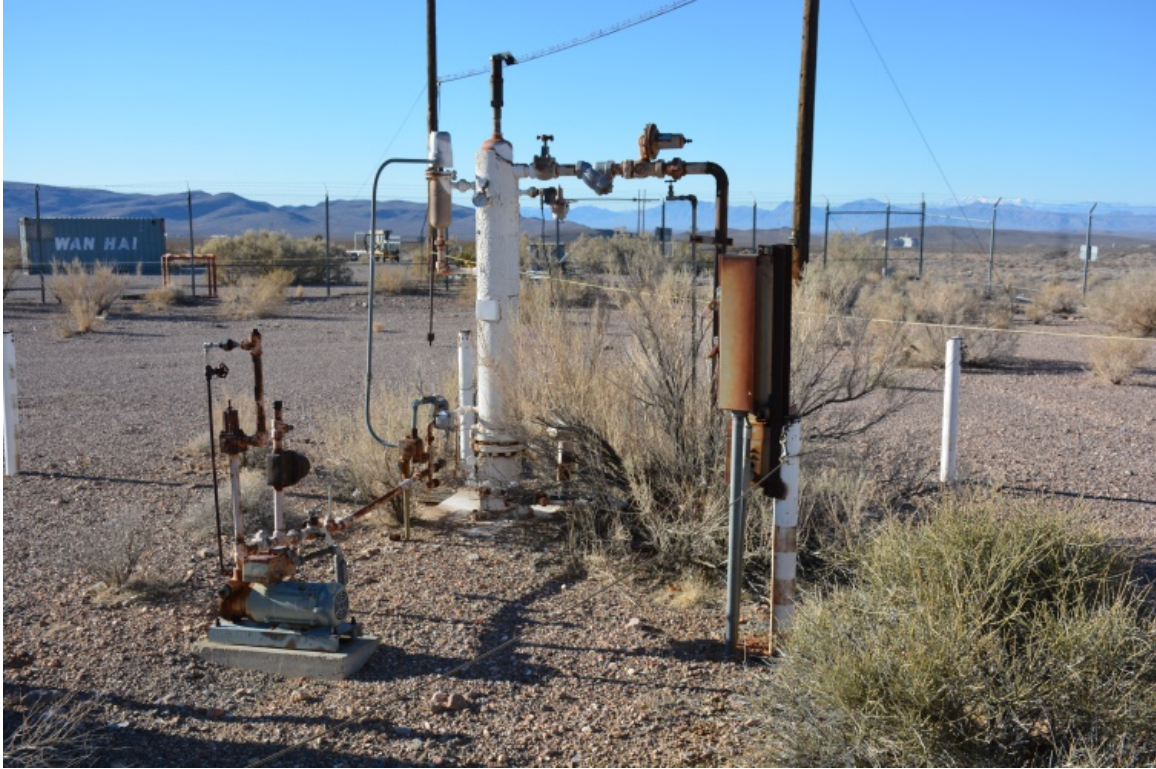
Figure 57. AR-3 (25-3220), manifolds, valves, regulators, and other Propane Storage Area related equipment mounted on small concrete pads, facing southwest (DRI 2019, Photo 380).
