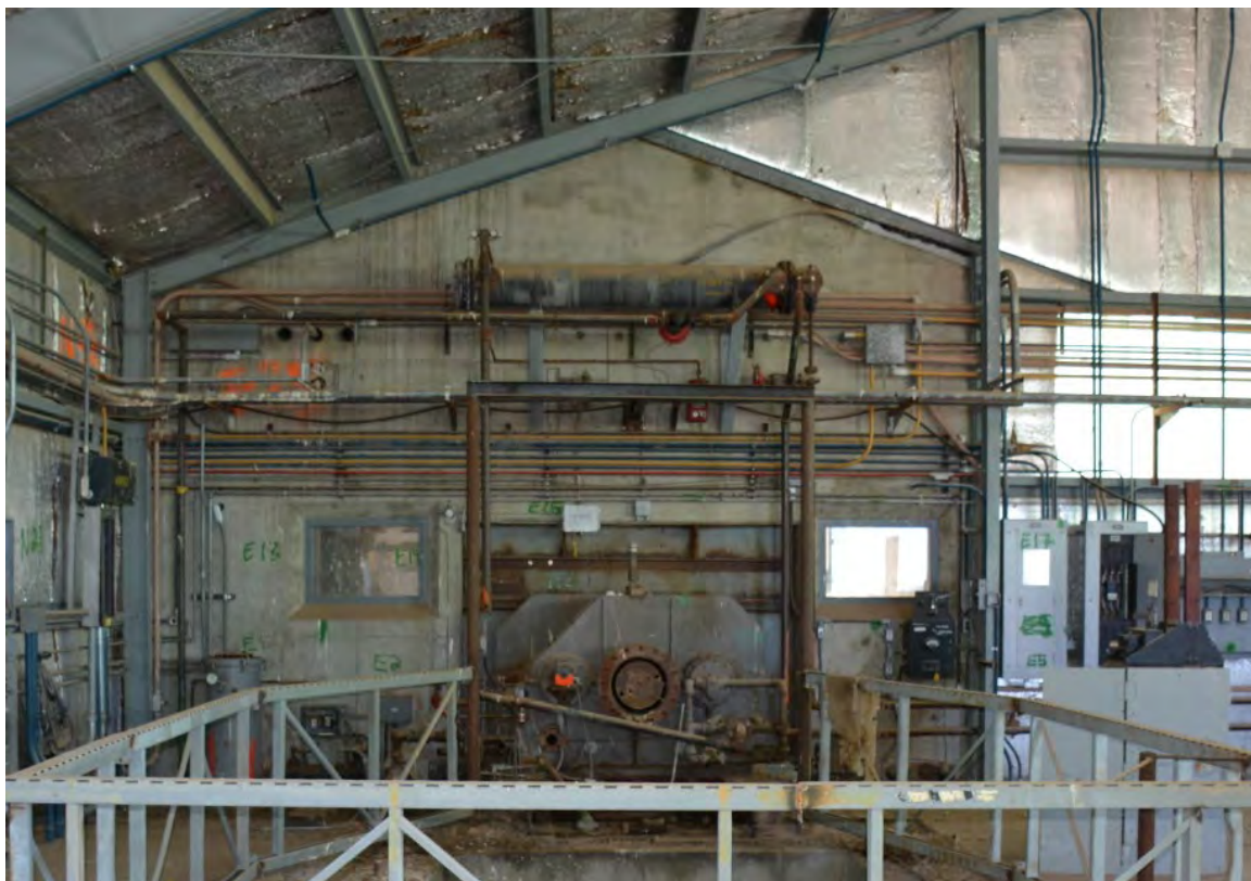
South portion of concrete west elevation of Cryogenic Pump Building visible from inside the Motor Drive Building. Drive shaft at center extends into the Cryogenic Pump Room (DRI, Photo 954, 2019).
