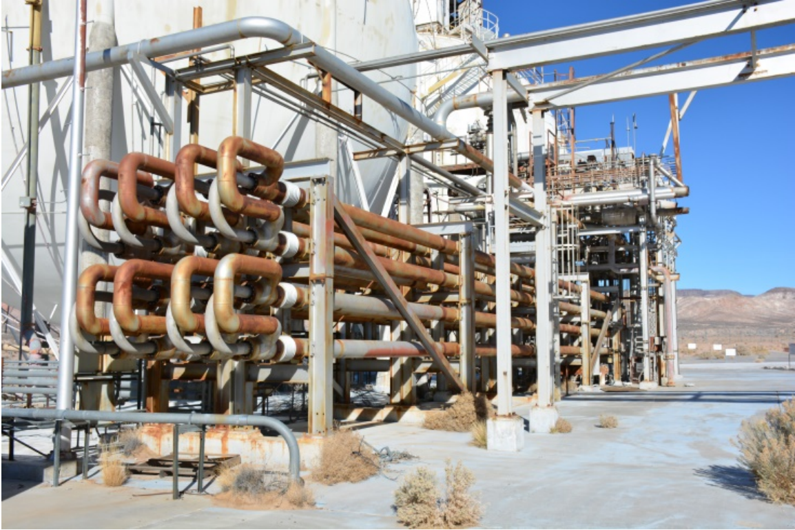
Figure 26. AR-3218C (25-3210), current detail of expansion joints of the Turbine Energy Source/Exchanger, facing northwest (DRI 2019, Photo 486).
