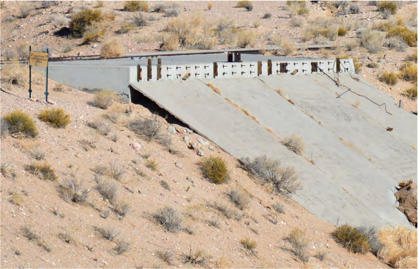
A zoomed in view of the test stand from the image on the first page (DRI, Photo 202, 2019). The yellow sign on the left indicates that the pad is a contamination area.
