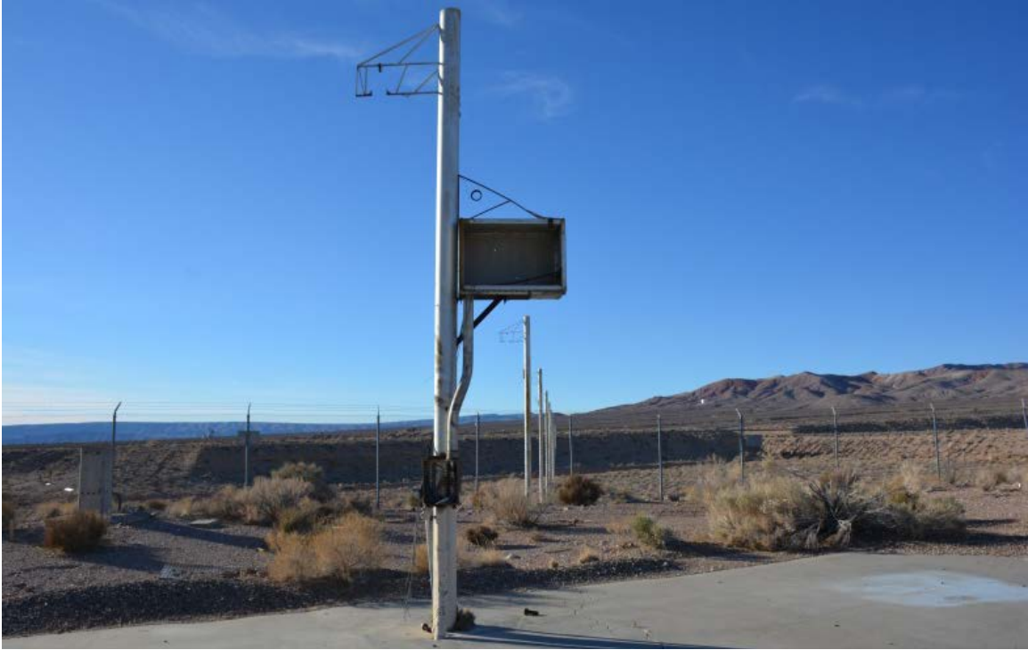
Figure 28. AR-6 (25-3210), Dosage Measurement Aerial Trolley, poles across Topopah Wash, facing northwest. Nearest pole inside the perimeter fence has trolley bracket at top and communications/ electronic lines below (DRI 2019, Photo 372).
