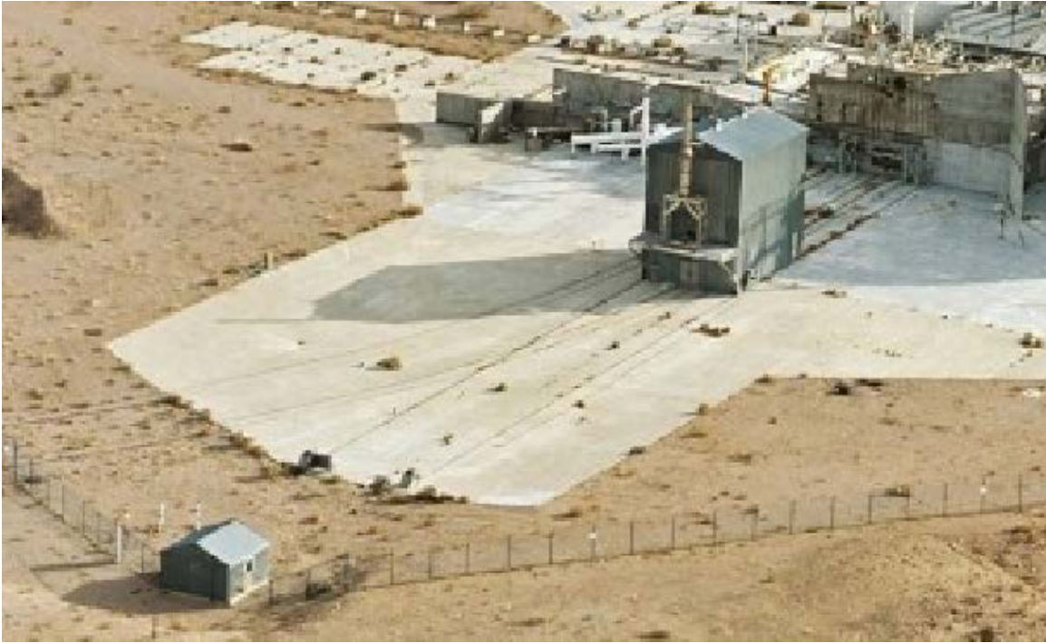
Figure 41. Reactor Shed Funicular Railroad, facing southeast (Detail, RSL 2000). Two phases of slab construction are evident. Both gabled buildings have been demolished.
