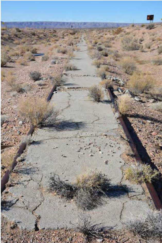
Concrete-filled railroad bed (AR-1) east of Test Stand, facing west. Photo is taken from the eastern terminus of the altered section of track (DRI, Photo 113, 2019).
