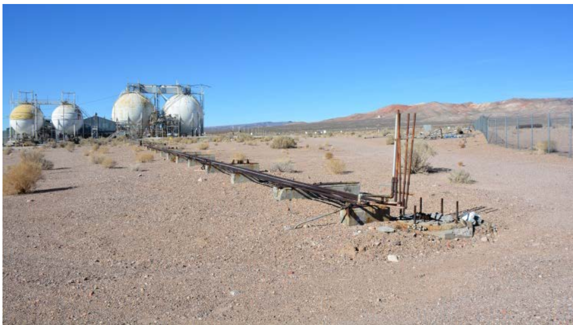
Figure 34. AR-19 (25-3210), skeletal steel supports and concrete piers, remnants at the east end of the flume and Flare Stack footer shown above (DRI 2019, Photo 564).
