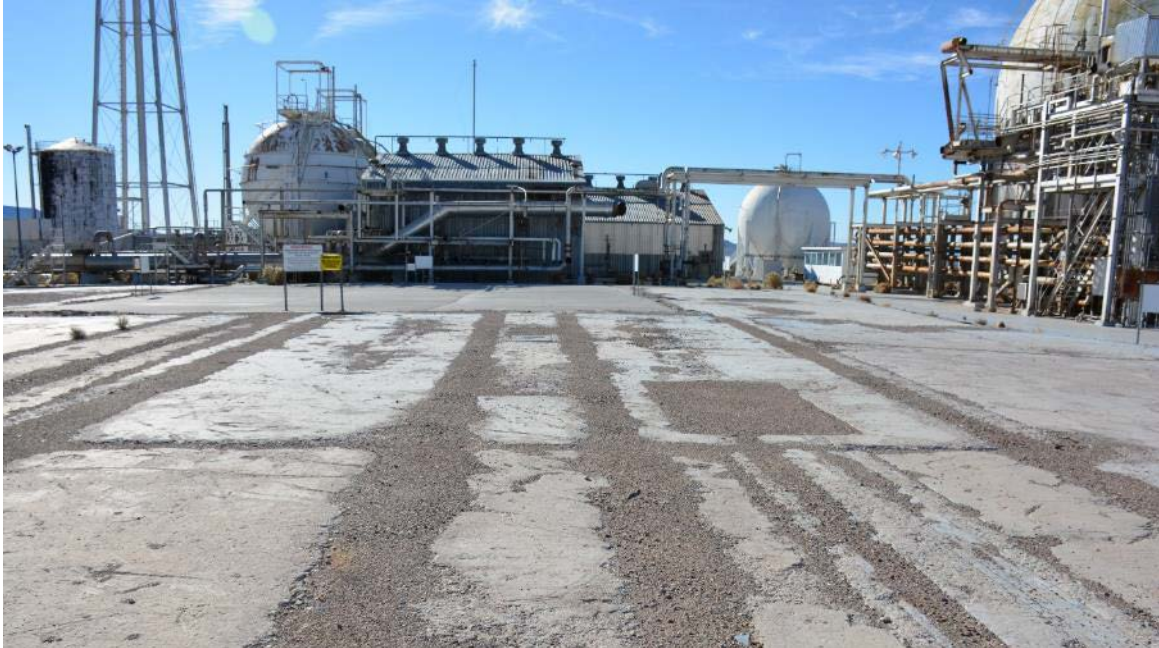
Figure 22. Remnant foundation and gravel-filled rail paths of 25-3210/AR-3206, the Reactor Pad (DRI 2019, Photo 458).
