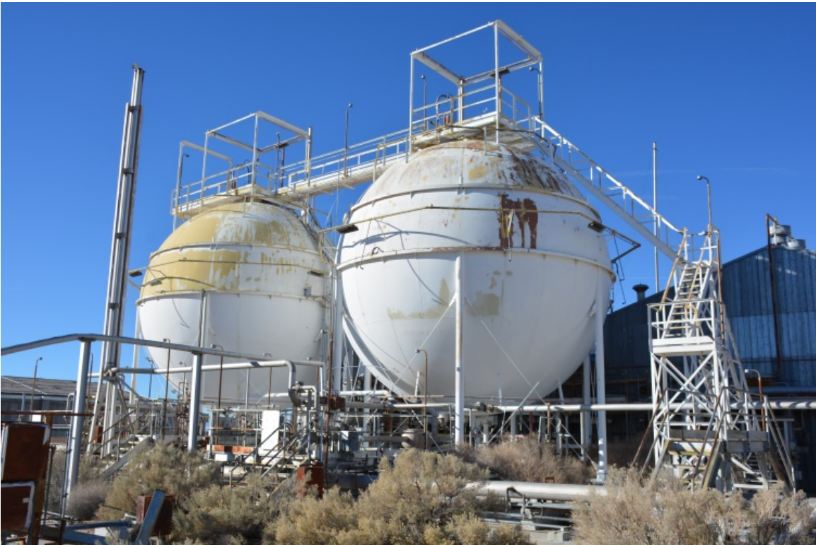
Figure 74. AR-3213 (25-3230-32), Liquid Hydrogen (LH 2 ) Dewars 4 and 5, facing southwest (DRI 2019, Photo 426).
