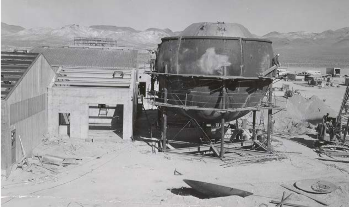
Figure 73. This photo of Dewar 4, 25-3230-32/AR-3213 under construction shows its double-wall construction (REECo 1960, Photo 888-10).
