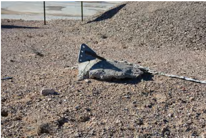
AR-22, grounded anchor for upper four northwest guy cables (DRI 2019).
