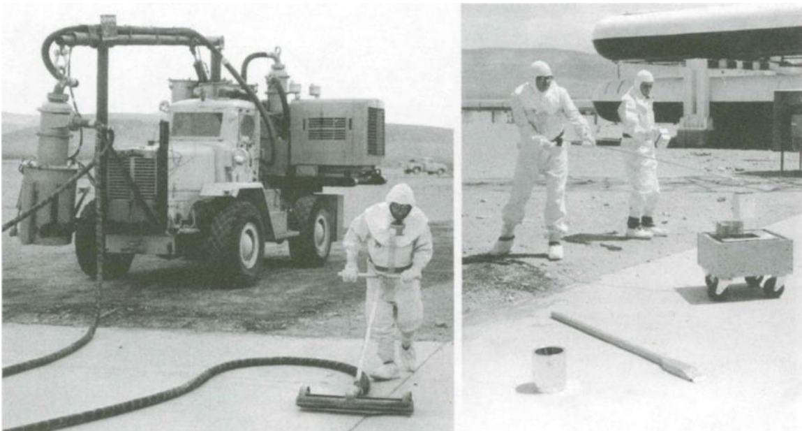
Figure 88. Manual decontamination at Test Cell C using a truck-mounted vacuum and a lead-shielded dolly (photographer: Los Alamos Scientific Laboratory, reproduced from Dewar 2004:130).
