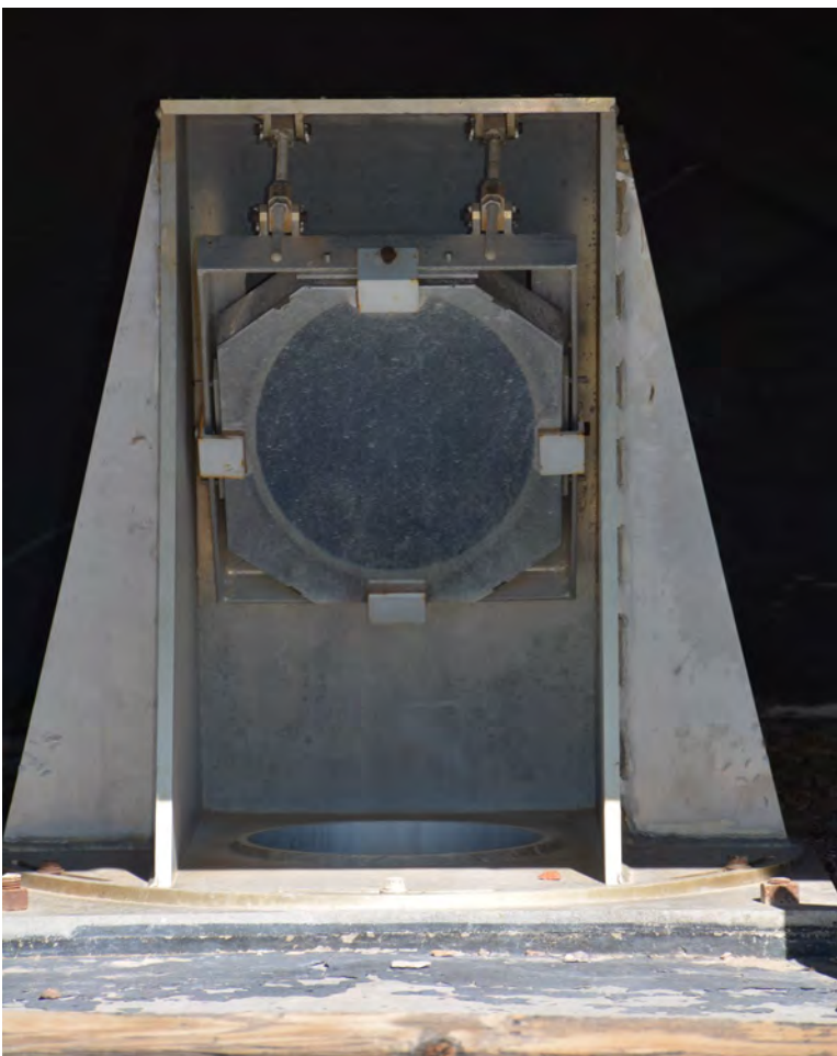
Detail of periscope from outside building with mirror in place (DRI, Photo 158, 2019).
