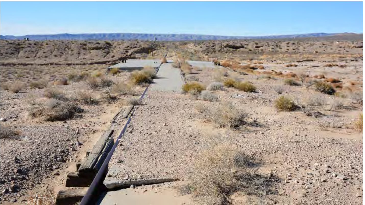
Test Stand on causeway over Topopah Wash, facing west. Concrete-filled railroad bed (AR-1) is in foreground (DRI, Photo 164, 2019).
