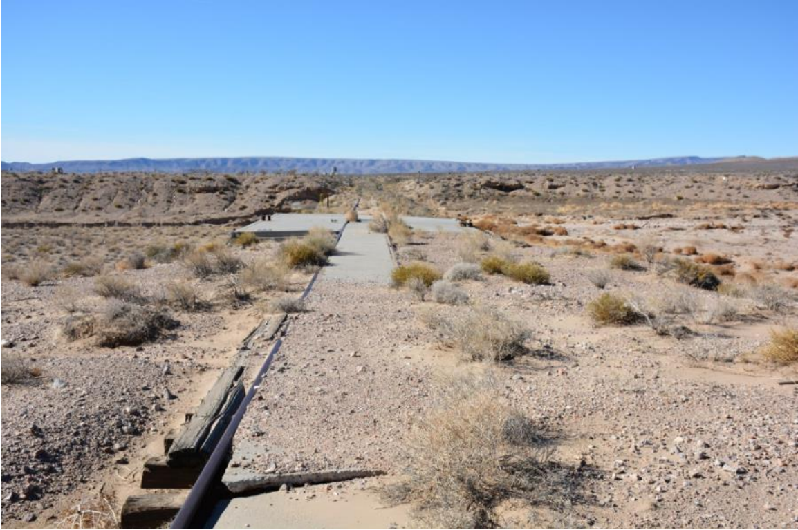
Figure 83. The Kiwi-TNT Reactor Test Stand on causeway over Topopah Wash, facing west. Concrete-filled railroad bed (AR-1) is in foreground (DRI 2019, Photo 164).
