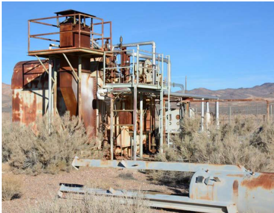
Figure 56. AR-1 (25-3220), Process Water Heater, facing northwest. The base of the once vertical Water Conditioner (AR-2) is in the foreground (DRI 2019, Photo 378).
