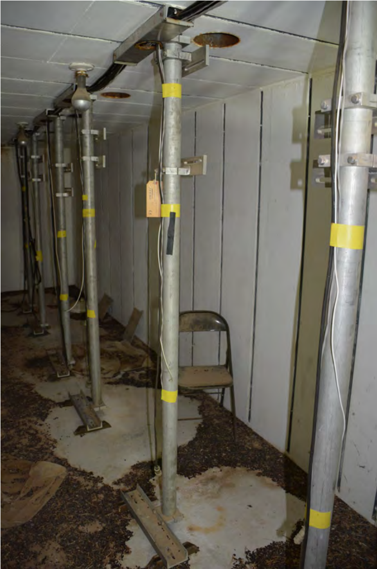
Oblique view of periscope poles, note viewing ports in ceiling by each pole, facing southeast (DRI, Photo 1096, 2019).
