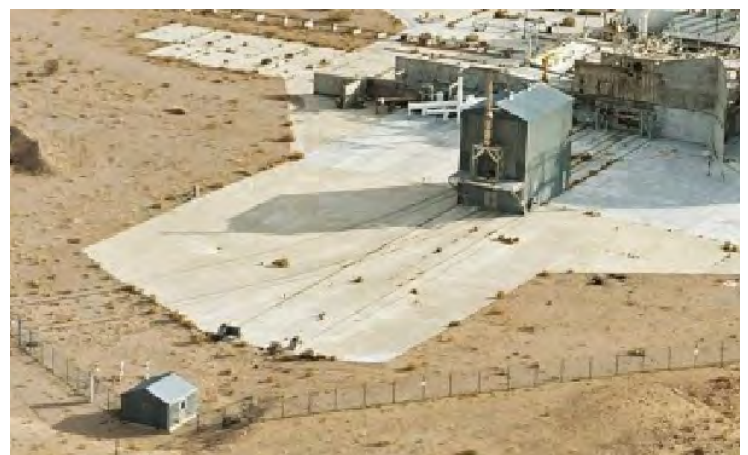
Reactor Shed Funicular Railroad, facing southeast (Detail, RSL, c. 2000). Two phases of slab construction are evident. Both gabled buildings have been demolished.
