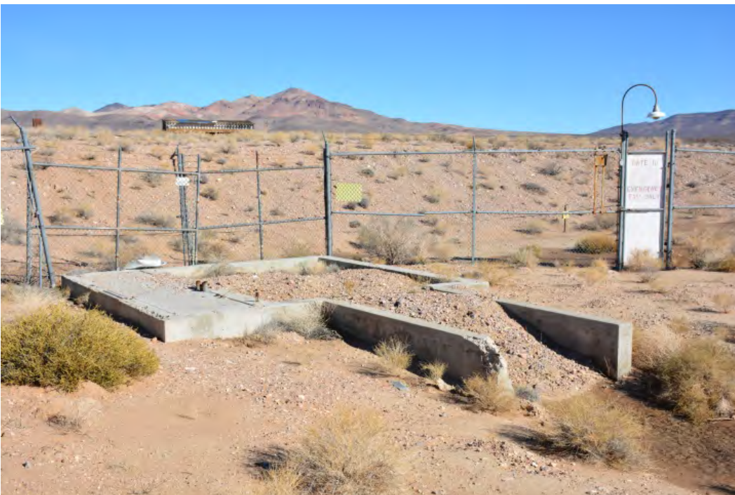
Elevation: N/A Direction facing: Northeast Photographer: DRI (Photo 516) Date: 2019 Shed Drive building foundation. Cable trench is at right in foreground.
