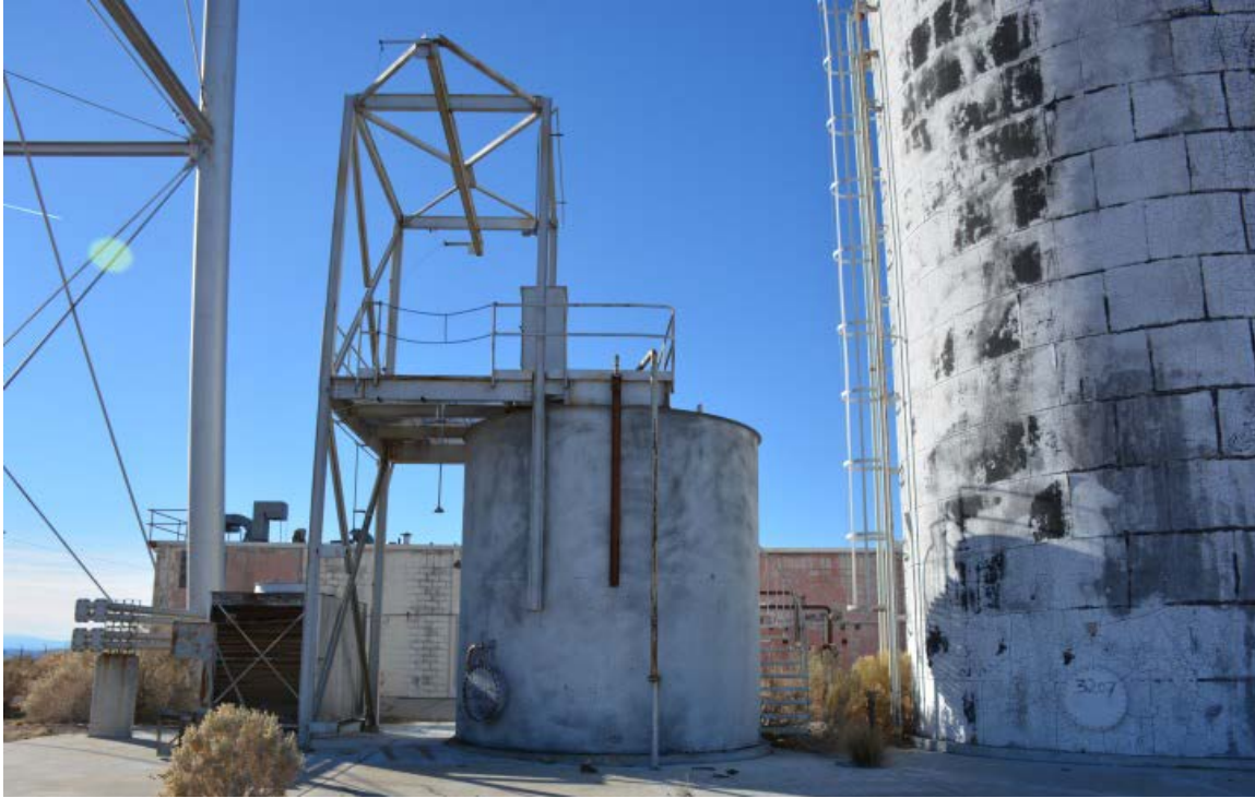
Figure 49. AR-3207 (25-3220), Mixing Tank with overhead crane for Borated Water System, facing west (DRI 2019, Photo 288).
