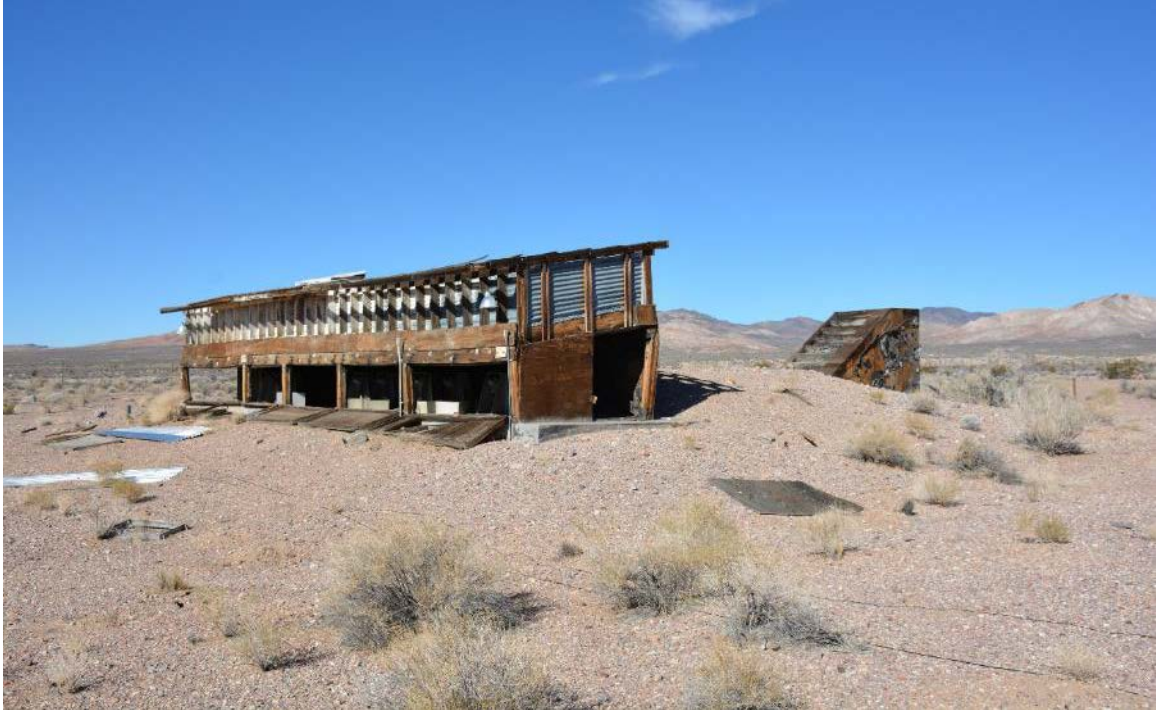
Figure 59. AR-3226, overview of the North Camera Bunker, facing northwest (DRI 2019, Photo 116). Visible on the surface are the Periscope Gallery (left), Entry Shed (right), and Berm.
