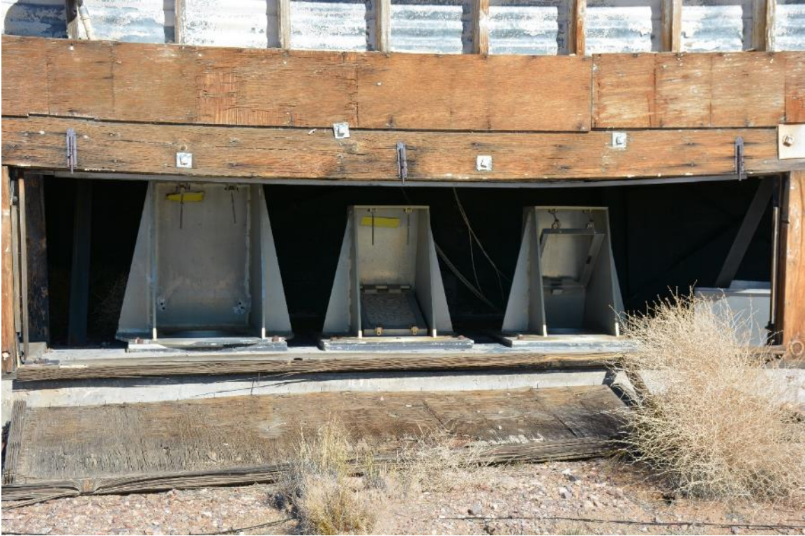
Figure 61. AR-3226, detail of periscopes in westernmost bay of the North Camera Bunker (DRI 2019, Photo 154).
