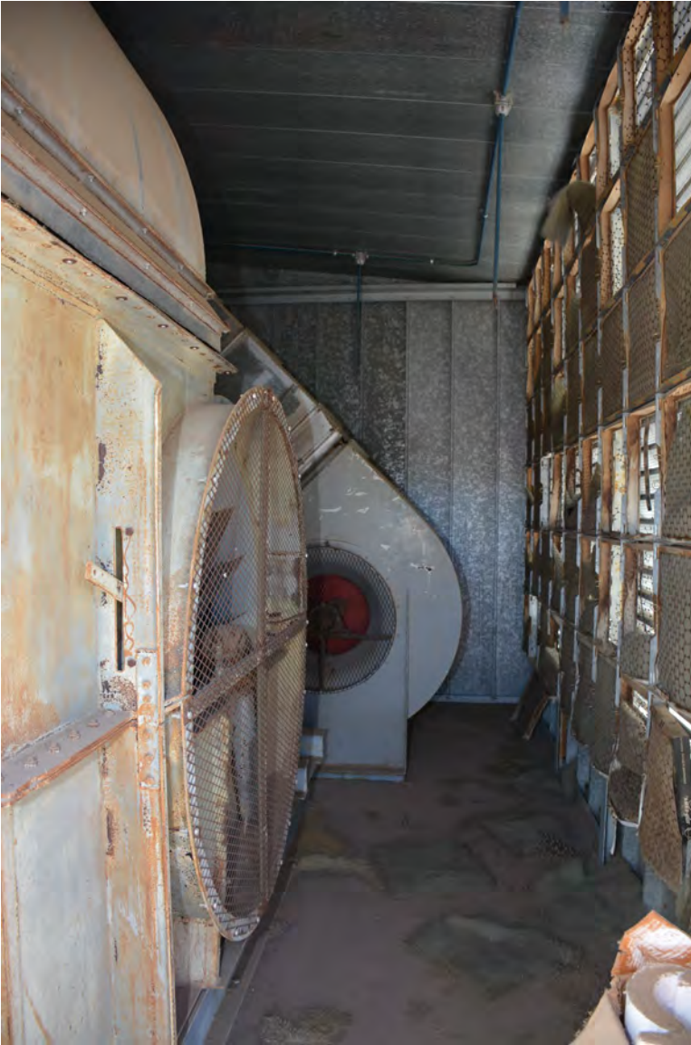
Blowers and filter panels in Filter Room of Motor Drive Building (DRI, Photo 984, 2019).
