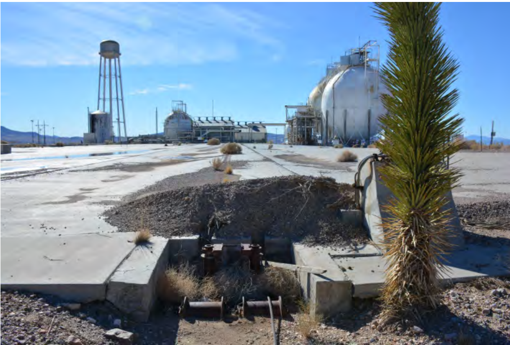
Cable guide rollers and stop block at the north end of the TCC Facility concrete foundation, facing south (DRI, Photo 508, 2019).
