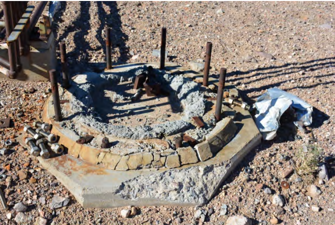
Detail of Flare Stack Foundation (DRI 2019).
