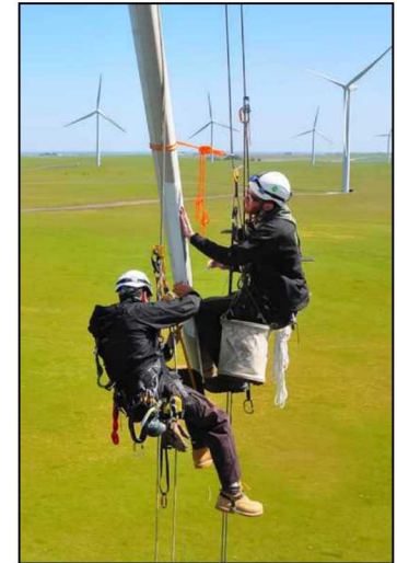
Scarfed Blade Repair Process
