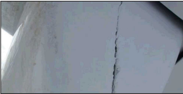
Severe Growth of Fiber Fracture
