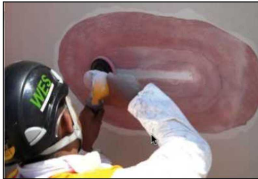
Scarfed Blade Repair Process
