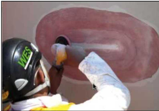
Scarfed Blade Repair Process
