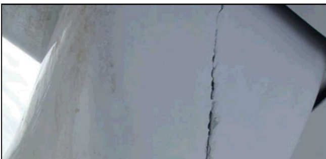
Severe Growth of Fiber Fracture
