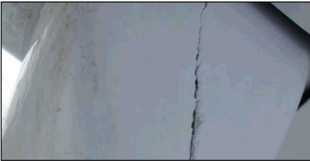
Severe Growth of Fiber Fracture
