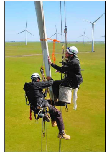
Scarfed Blade Repair Process
