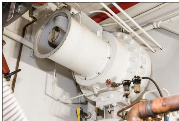
Heavy cast-iron exhaust air outlet in the northwest corner of the room (DSC2318).
