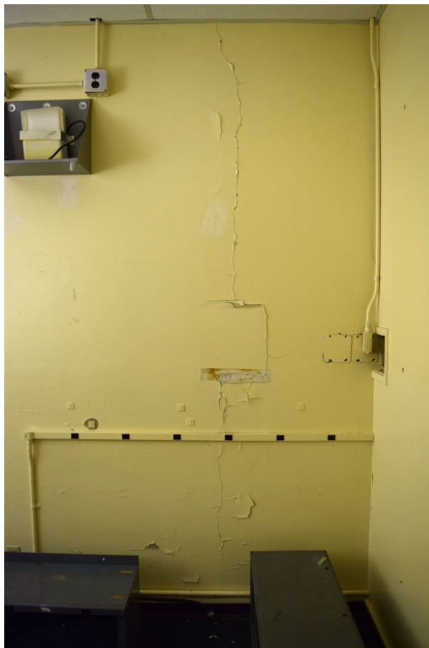
Figure 206. Crack completely through concrete in south wall of CP-1, Room 241B (2016).
