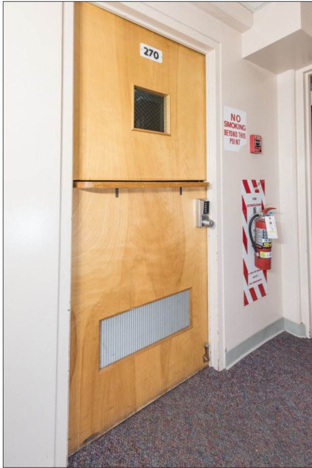
Figure 183. Typical interior Dutch door was often used to keep people out of spaces while allowing free communication through the open top panel. This door is also equipped with a combination lock. Small reinforced windows are also common to allow identification of visitors before opening the door (photograph DSC2118 dated 2016 on file at RSL).
