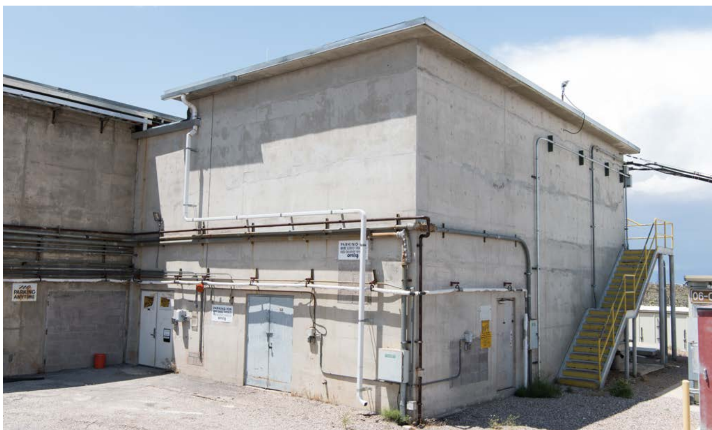
Figure 98. South and east façades of CP-1A. Pour lines are highly visible in this view (photograph DSC3330 dated 2016 on file at RSL).
