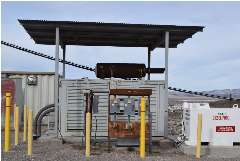
Figure 166. AR6 standby generator, canopy, and fuel tank (2016).
