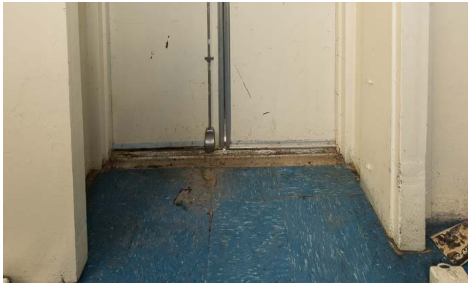
Figure 218. Silt and floor damage from water entering west door of CP-1B (photograph DSC_2524 dated 2016 on file at RSL).
