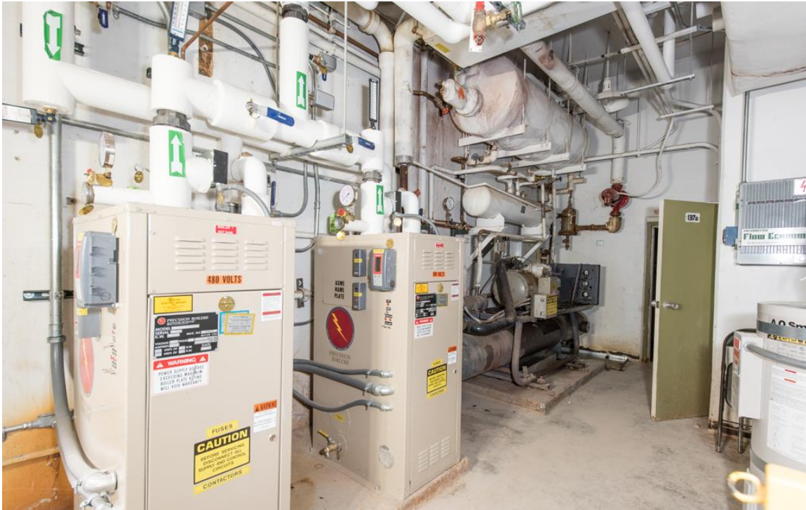
Electrical boilers and chiller in Room 137. (NSTec DSC2327, 5/2/2016)
