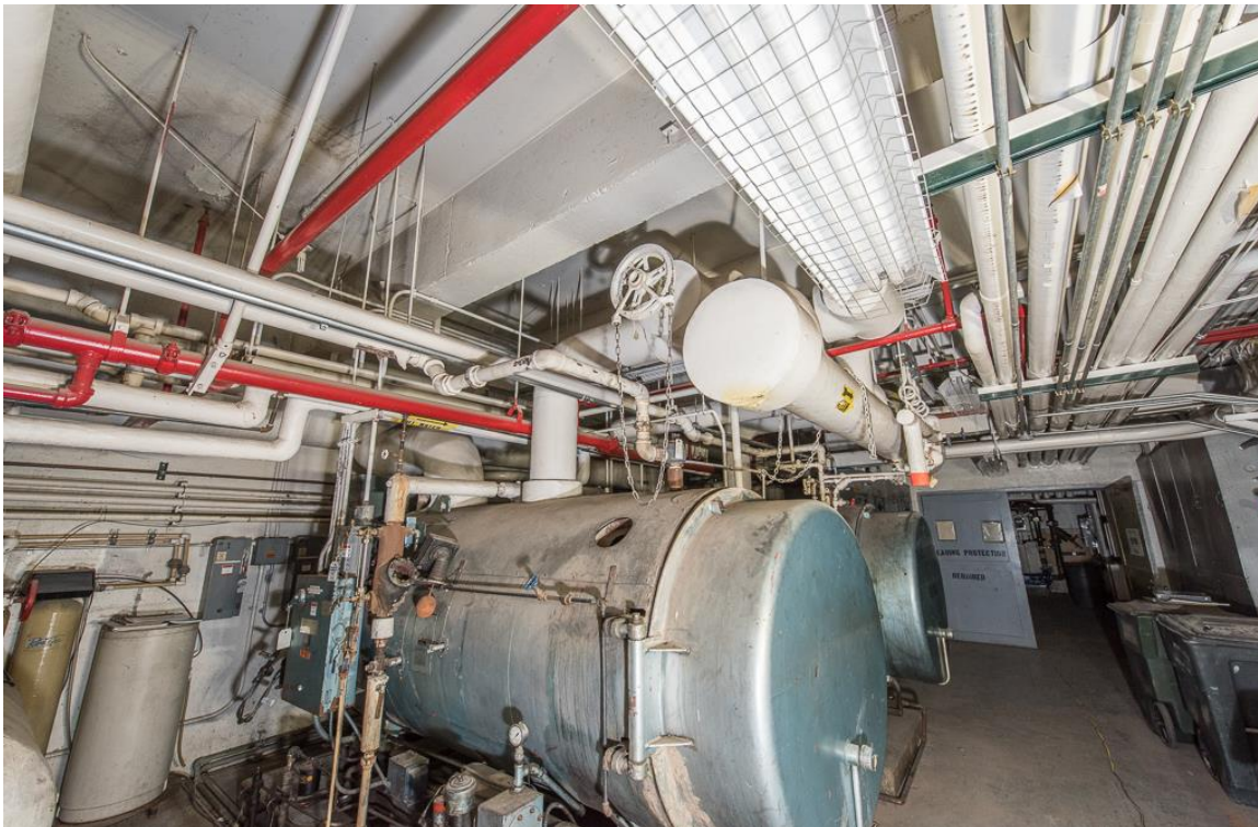
Diesel-fueled boilers in Room 117. (NSTec DSC2969, 5/5/2016)
