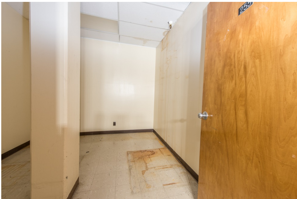
Figure 214. Water damage in ceiling, wall, and floor from ceiling leak in Room 255 (photograph DSC1612 dated 2016 on file at RSL).
