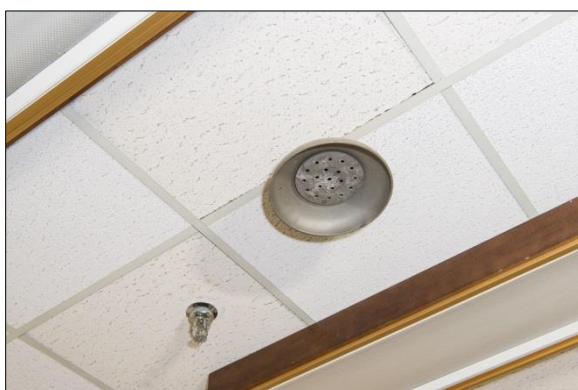
Decontamination shower head (DSC3001).
