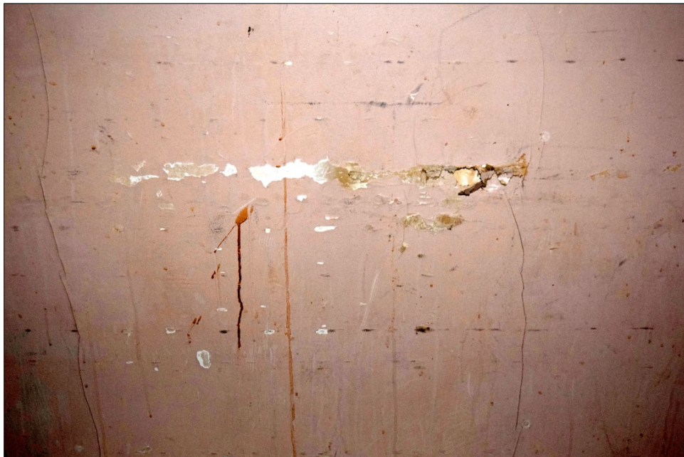
Figure 221. Wall damage caused by kitchen carts in CP-1 basement corridor. Also visible are vertical cracks likely from seismic activity (2016).
