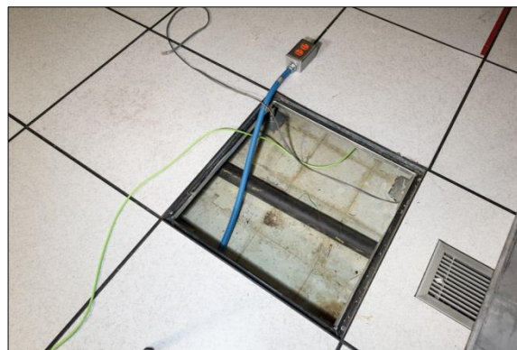
Raised floor with panel removed, showing original floor of light green tile (DSC2666).
