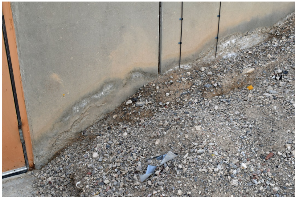
Figure 210. Erosion of exterior concrete at CP-1B. No waterproofing is visible (2016).
