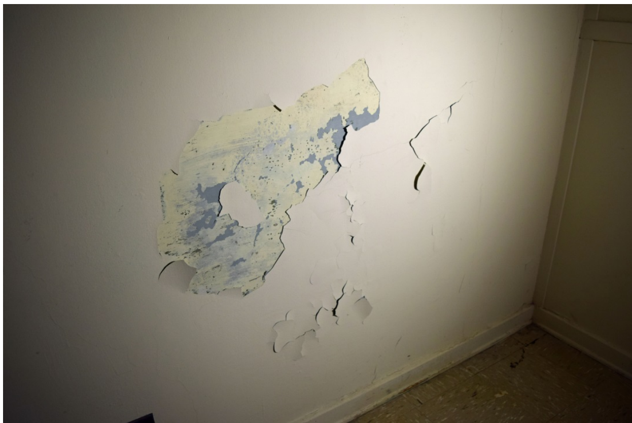
Figure 219. Failure of paint to adhere to concrete, interior of south wall, CP-1 (2016).
