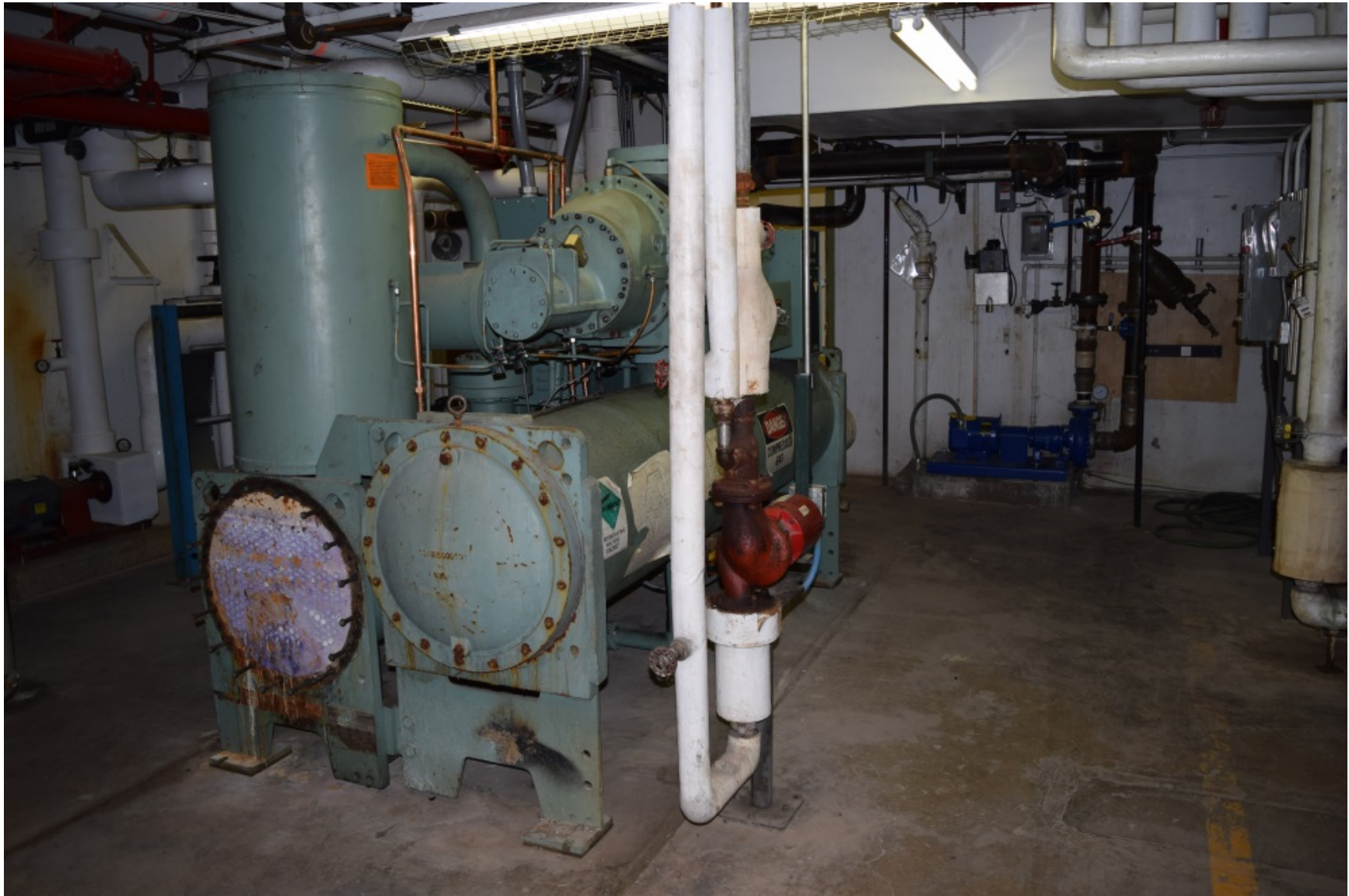
Figure 224. Broken CP-1 chiller in Room 116 with end removed (2016).
