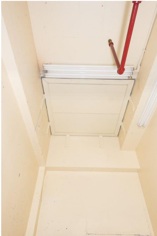
At left is ceiling plug in Room 101A after removal of spiral staircase and at right is the CP-1B staircase. (NSTec DSC2153, 5/2/2016; DSC2835, 5/5/2016)
