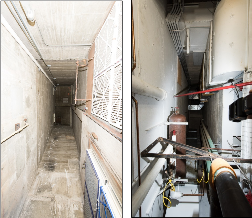
Figure 137. Views upward into the CP-1 air intake and exhaust ducts (photographs DSC2942 and DSC2983 dated 2016 on file at RSL).
