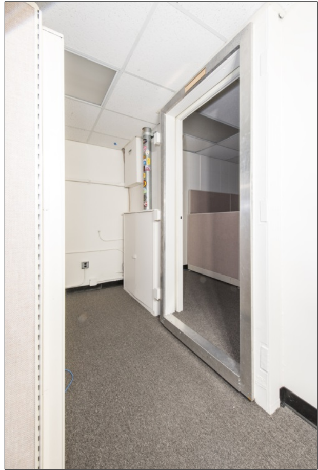
Figure 184. Vault. Although the door has been removed from Room 272, the massive steel frame indicates that this was one of the higher-security vaults with steel and concrete walls (photograph DSC2105 dated 2016 on file at RSL).
