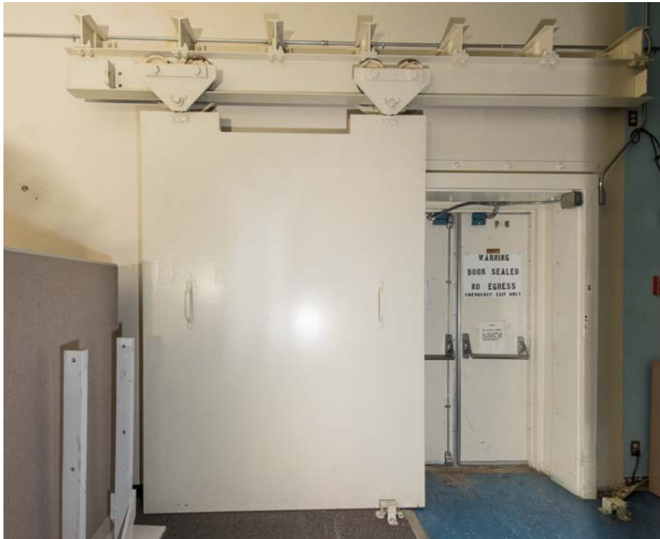
Figure 176. Lead-shielded blast door at west entrance to CP-1B (photograph DSC2523 dated 2016 on file at RSL).
