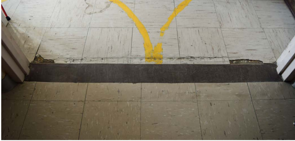
Figure 201. Cracking of concrete and tile at junction of CP-1 and CP-1B visible in main entrance lobby, Room 205 (2016).
