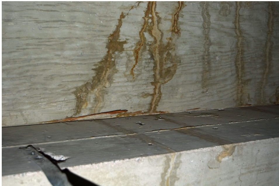
Figure 207. Water infiltration through ceiling cracks in CP-1 above Room 215 (2016).
