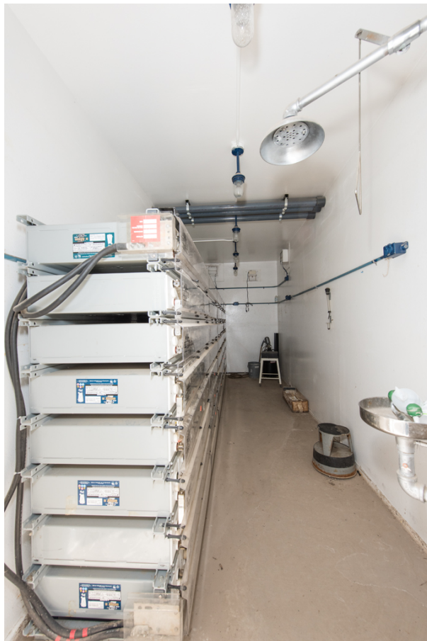
Figure 164. AR4 UPS Battery Room from entrance (photograph DSC2706 dated 2016 on file at RSL).
