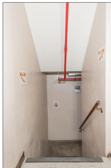
Stairs down from the first floor to landing, fire water main suspended from the ceiling, view south (DSC2208).
