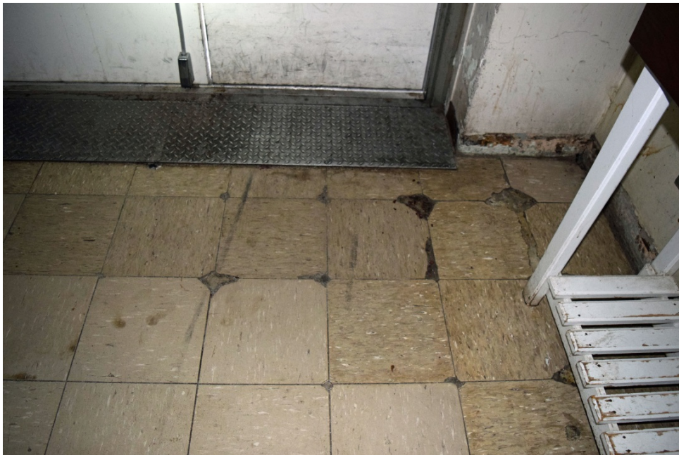
Figure 202. Cracking of concrete and tile at junction of CP-1 and CP-1A visible in basement entrance, Room 115A. Also present is baseboard damage from minor flooding through doorway and heavy use wear. Note at least two earlier generations of tile replacements from older damage. Light is also visible through door, indicating a route of insect and possibly mouse access (2016).
