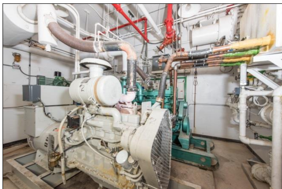
View from the door showing emergency generators (n=2), compressor, blast exhaust, fire suppression, view southwest (DSC2304).
