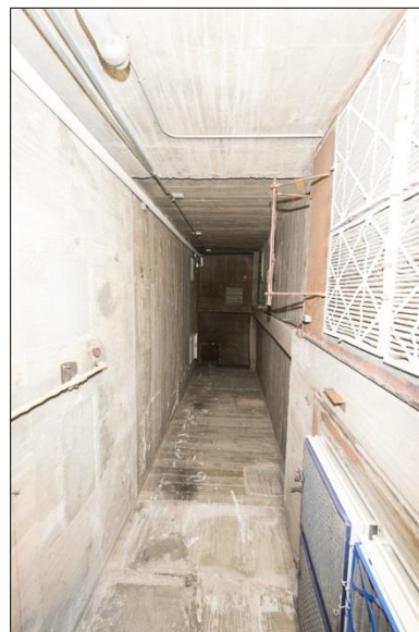
View of air intake and plenum upward to the roof as 256A (DSC2942).
