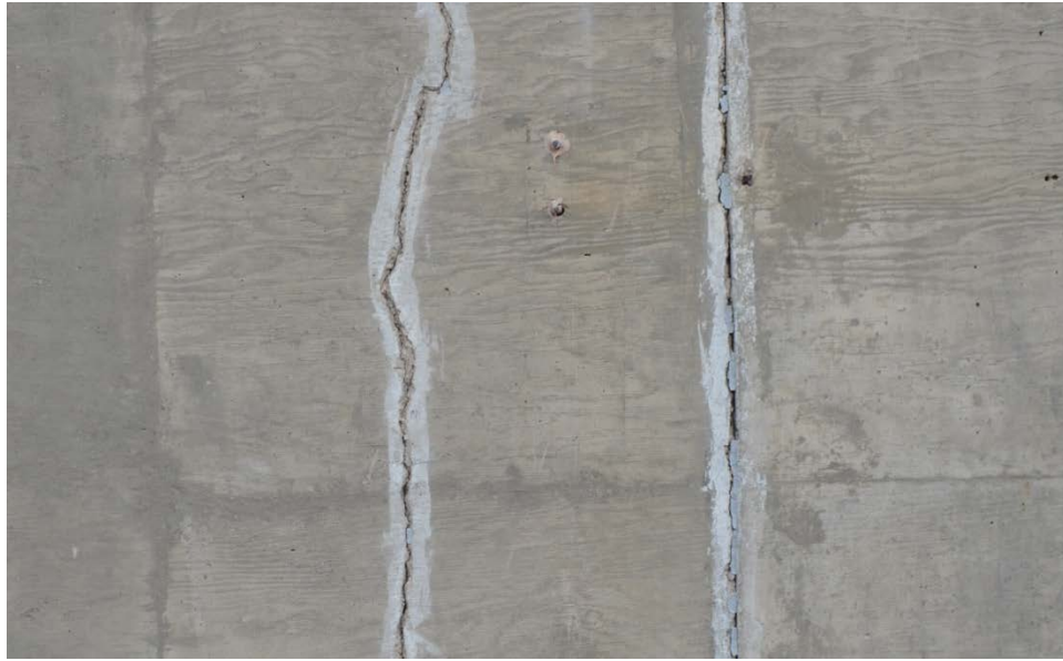
Figure 205. Detail of CP-1 west wall cracks (2016).
