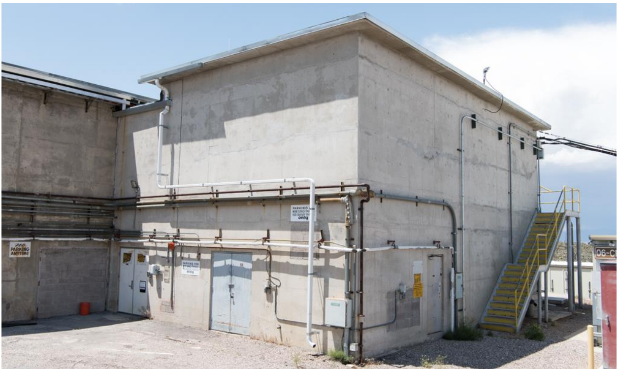
South and east façades of CP-1A, facing northwest. Pour lines are highly visible in this view. (NSTec DSC3330, 5/24/2016)
