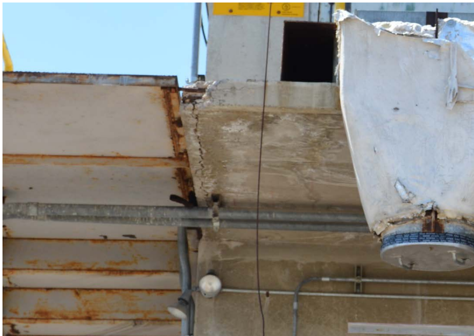
Figure 212. Concrete decay at edge of north porch on CP-1A with exposed rebar (2016).
