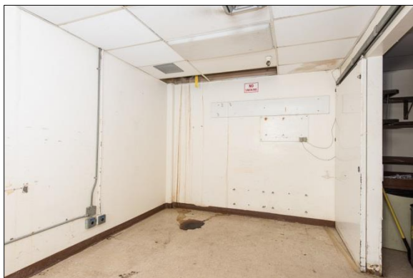
Western section of the room, note damage and leak from suspended ceiling, view southwest (DSC2912).
