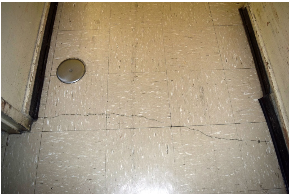
Figure 203. Crack in concrete basement corridor in CP-1. Also visible is wall and baseboard damage from kitchen carts (2016).
