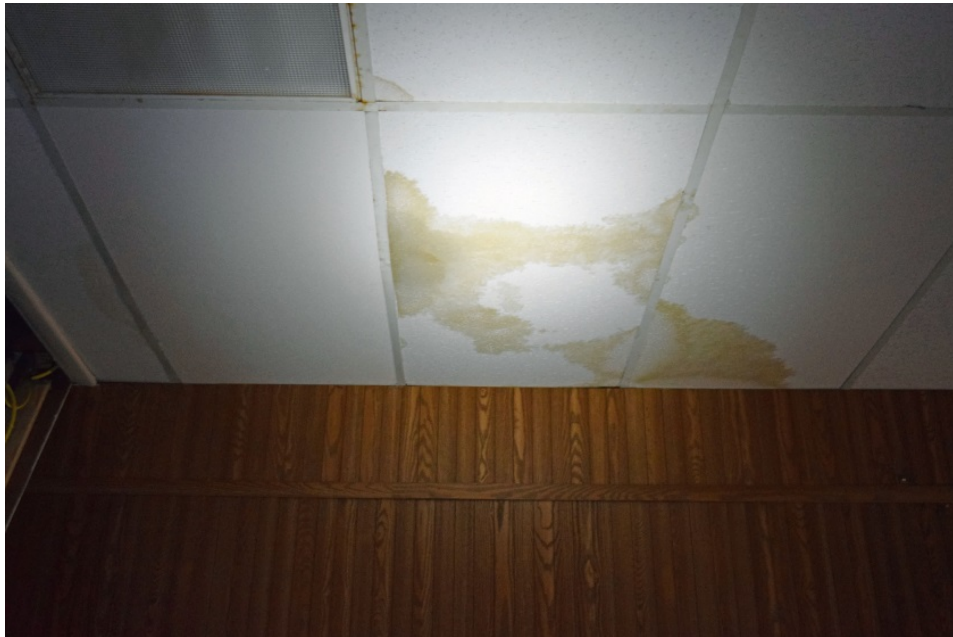
Figure 213. Water and possibly oil leakage onto ceiling of CP-1 Room 256 from air handler in attic (2016).
