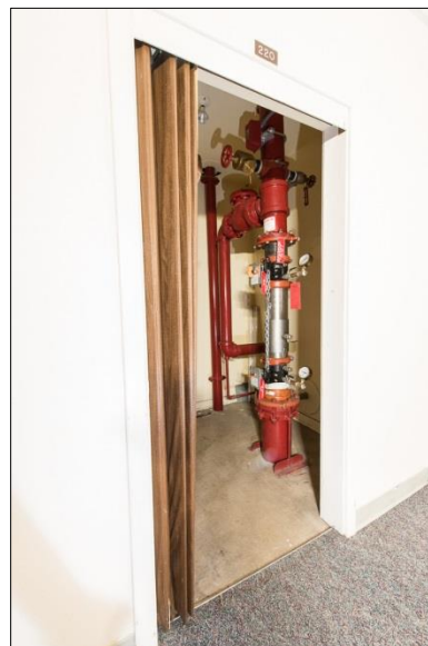
Fire main and valves in Room 220, view southwest (DSC1684).
