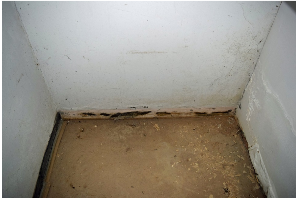
Figure 217. Silt accumulation, drywall damage, and baseboard failure in Room 137B. Again, water has entered through the basement door shown above (2016).
