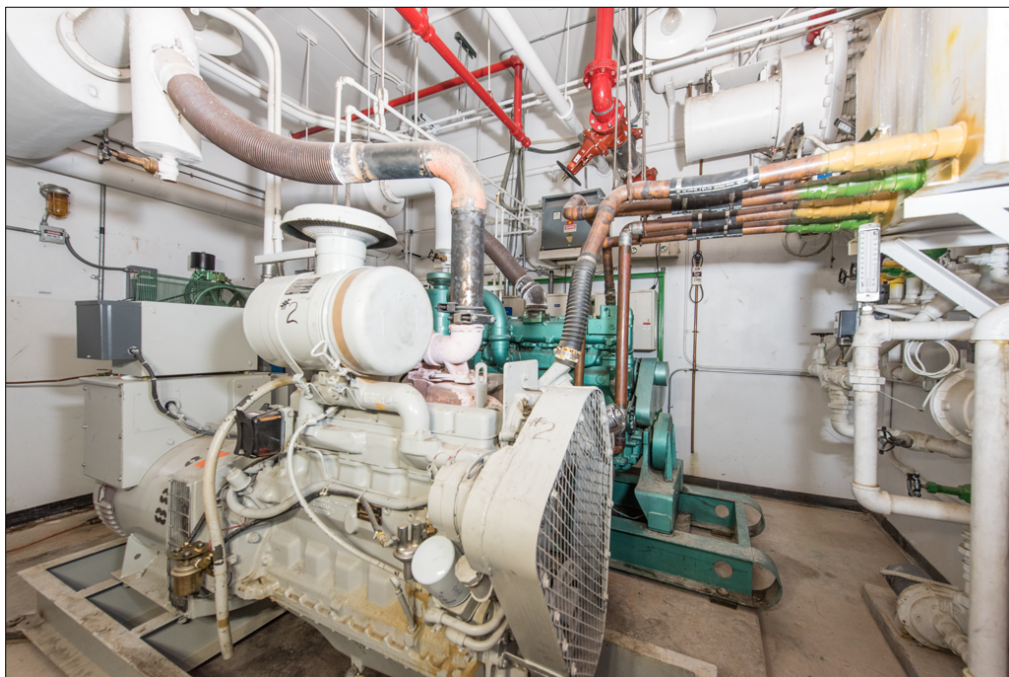
Figure 138. Emergency generators in Room 136 (photograph DSC2304 dated 2016 on file at RSL).
