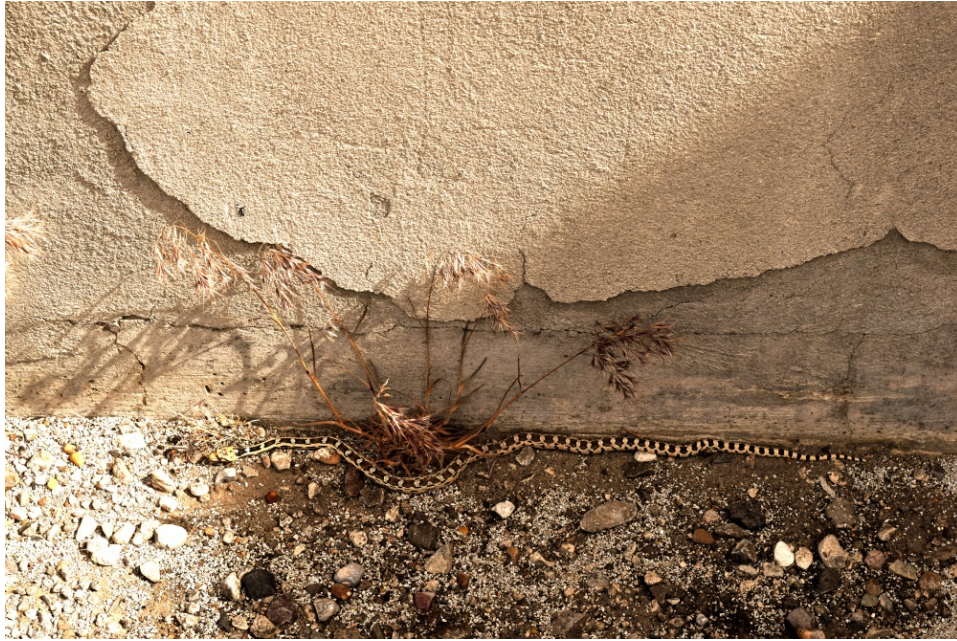
Figure 209. Erosion of stucco coating along foundation of CP-1B (2016).
