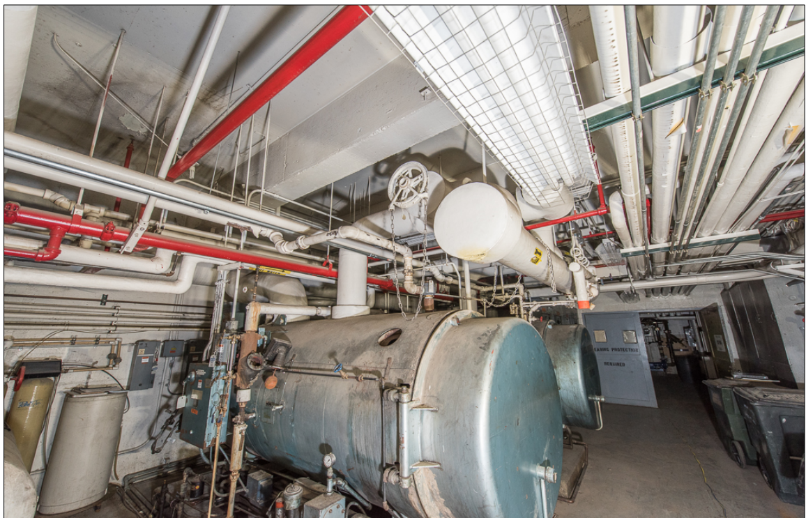
Figure 136. Diesel-fueled boilers in Room 117 (photograph DSC2969 dated 2016 on file at RSL).
