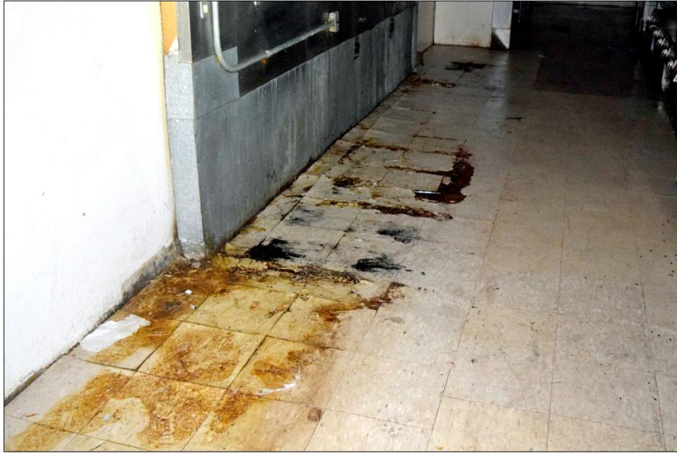
Figure 222. Floor damage below and behind removed equipment in Kitchen, CP-1 Room 112 (2016).
