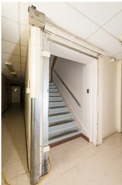
Figure 177. Overhead track and stop for blast door in basement of CP-1 (photograph DSC2614 dated 2016 on file at RSL).
