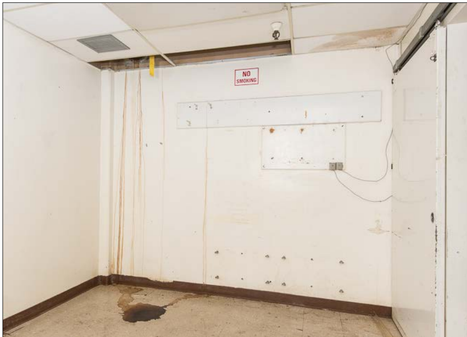
Figure 223. Kitchen grease flowing down wall and pooling on floor from vent due to removal of lower part of duct. Ceiling also has water damage (2016)
