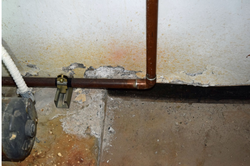
Figure 211. Exfoliation of concrete in basement Room 136 of CP-1B resulting from water infiltration through north foundation. This is the inside of the same wall shown above (2016).
