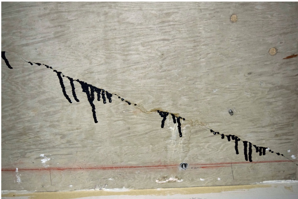
Figure 208. Tar and water infiltration through ceiling crack in CP-1 above Room 213 (2016).
