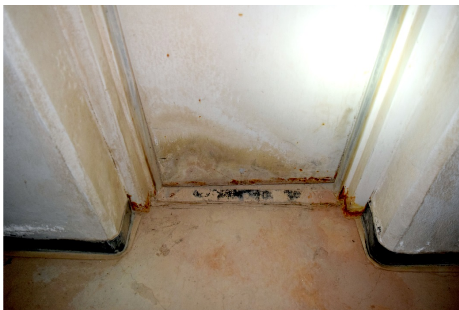
Figure 216. Silt accumulation and damage to steel door and frame to Room 137B from water entering through the door shown above and traversing entire length of Room 137 (2016).
