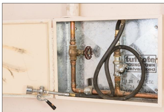
Hand-held sprayer mounted in box along west wall (DSC3011).
