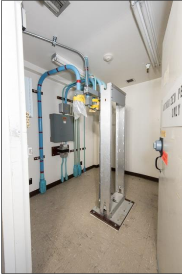
Interior view from entrance, Crypto Panel is mounted on the east wall, several cable conduits lead to the equipment rack, view southeast (DSC1978).
