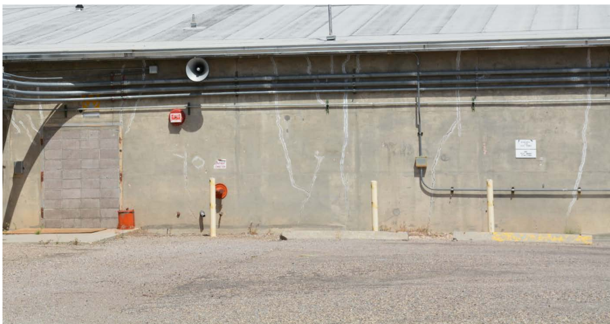
Figure 204. Wall cracks in west wall of CP-1 (2016).
