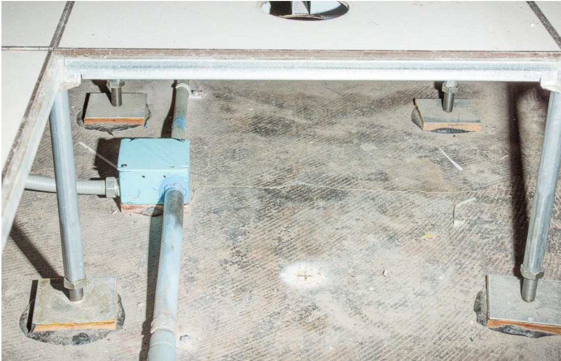
Raised computer floor system in Room 250 is typical of all others. (NSTec DSC1972, 4/20/2016)
