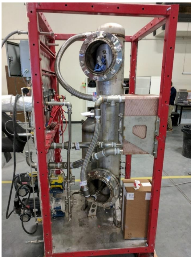
Figure 23. Spray tower during installation.
