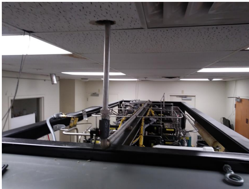
Figure 54-Relief header assembly, relief indicating sensor, and outlet plumbing that integrates to dilution duct above drop ceiling.
