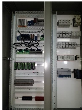
Figure 46. The electronics enclosure with the main components populated and awaiting field wiring to the instrumentation.
