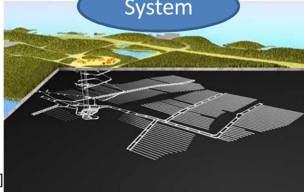
Canister and repository configuration
