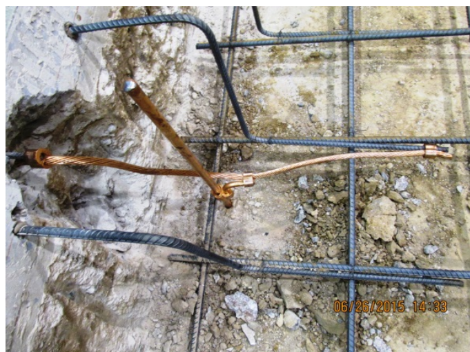
Figure 5: Grounding Cable and Rod
