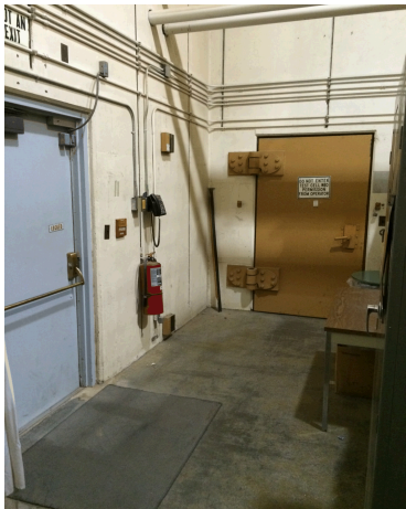
Photo 4: Standing just inside the interlocked gate. View of closed shield Door (Door A). Also the entrance door into the Test Cell
