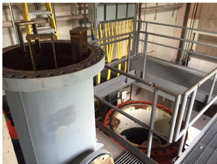
Figure 5.1-11. PFBC Pressure vessel bottom sections (red) and CHX2 (gray) in place.
