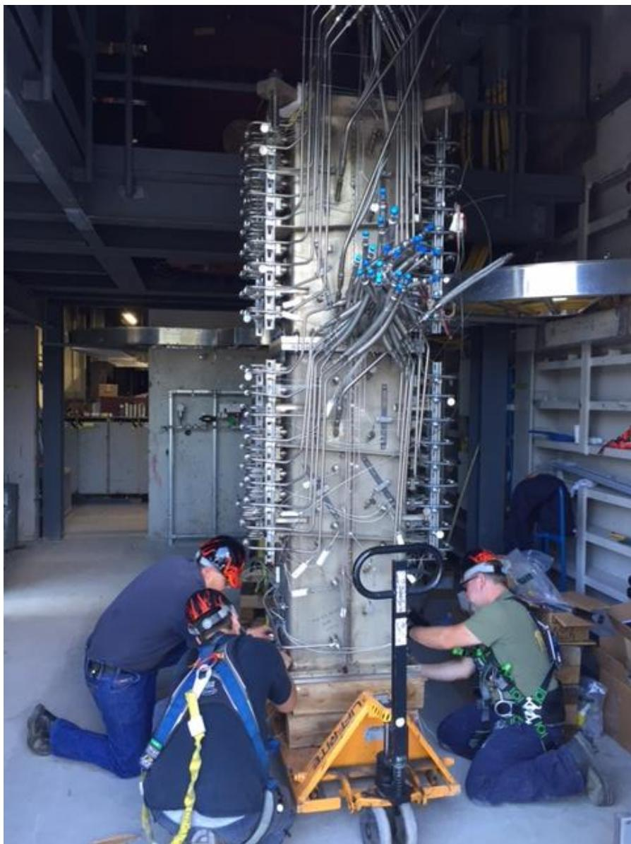
*Figure 5.1-9. Combustor sections assembled and ready to install.*
