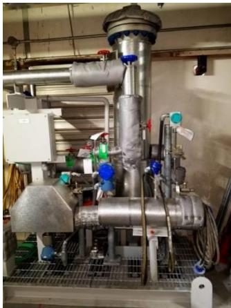
Figure 3-12: Module 4 with process condensate filter
