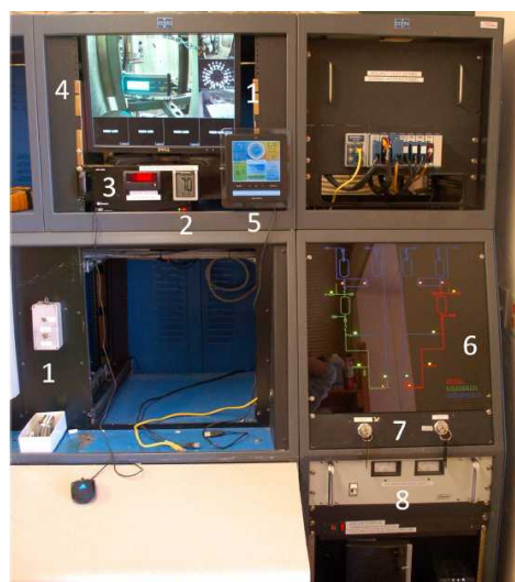
Figure 8: Console for operations and site monitoring. Visible are: Deadman's switch (1); Fuel galley temperature monitoring (2); Igniter supply voltage (3); Video observation system (4); Weather station (5); Valve status indicator panel (6); Propellant loading controls (7); and system power (8).
