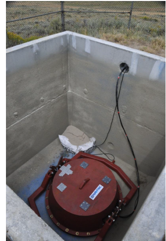
Figure 38 Dry Platform Photo
