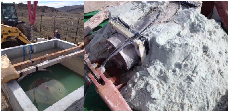
Figure 220 Wet Seafloor with Backfill Photo
