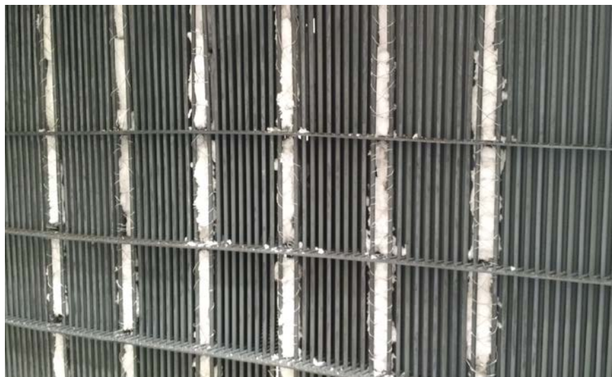
Figure 142: Heater Bundle with Insulation Installed in Gaps
