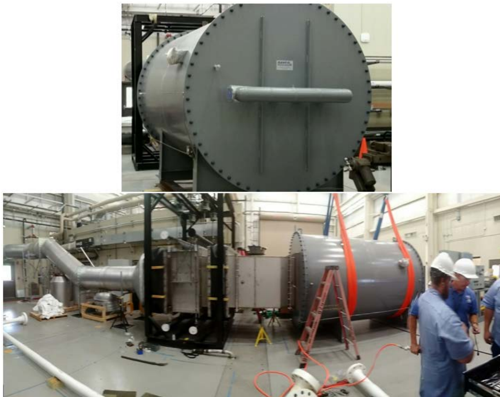
Figure 129: Gas Fired Primary Heater Installation
