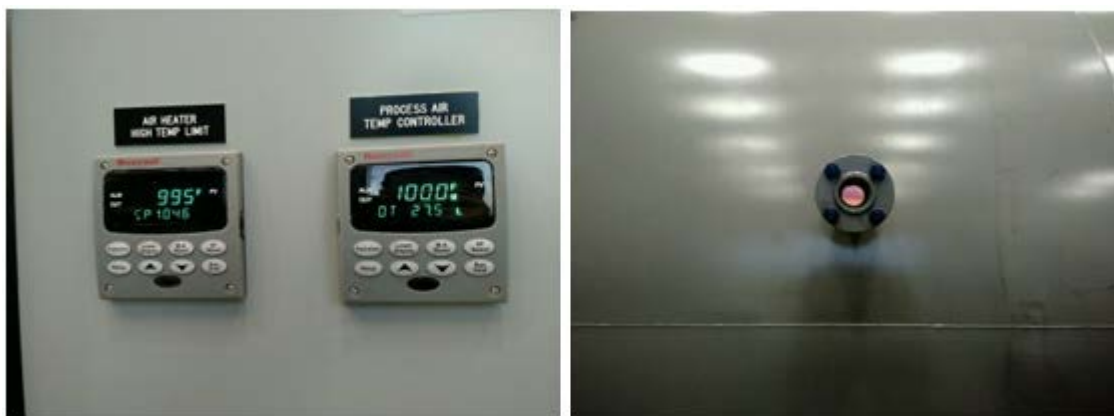
Figure 130: Commissioning Test of Primary Heater
