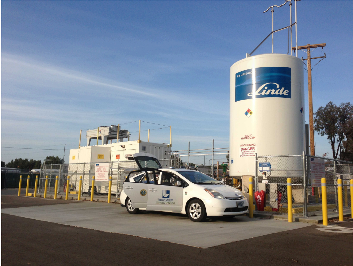
Figure 2. LLNL hydrogen experimental facility. The 345 bar 151 L cryogenic pressure vessel is installed onboard the Toyota Prius experimental vehicle [6]. The LH 2 pump is located inside the white container seen behind the back of the vehicle in this perspective, while the station Dewar for LH 2 storage is on the right.
