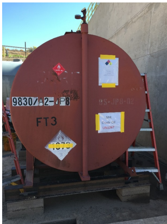
Figure F- 6: Unpressurized storage tank (~900 gal capacity) used to hold SPR oil from January – October 2018.
