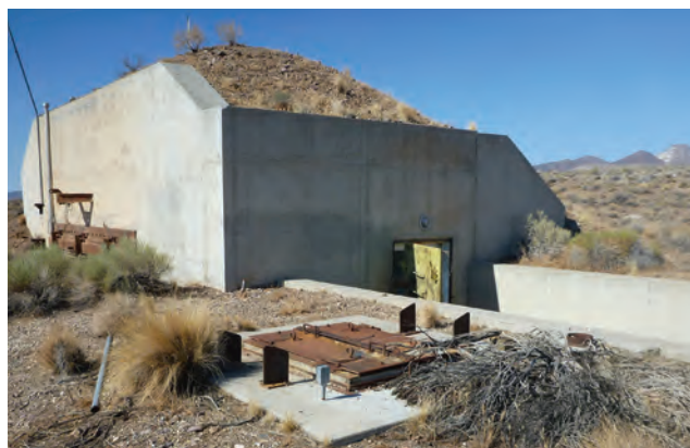
This Fast Photo Bunker for the Shasta test housed an ultra-high speed camera that recorded images of the nuclear detonation in microseconds.
