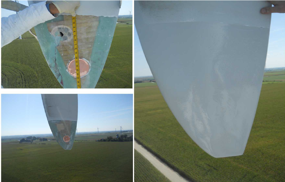
Figure 2-12: Picture of a Lightning Strike Tip Repair
