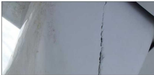
Severe Growth of Fiber Fracture
