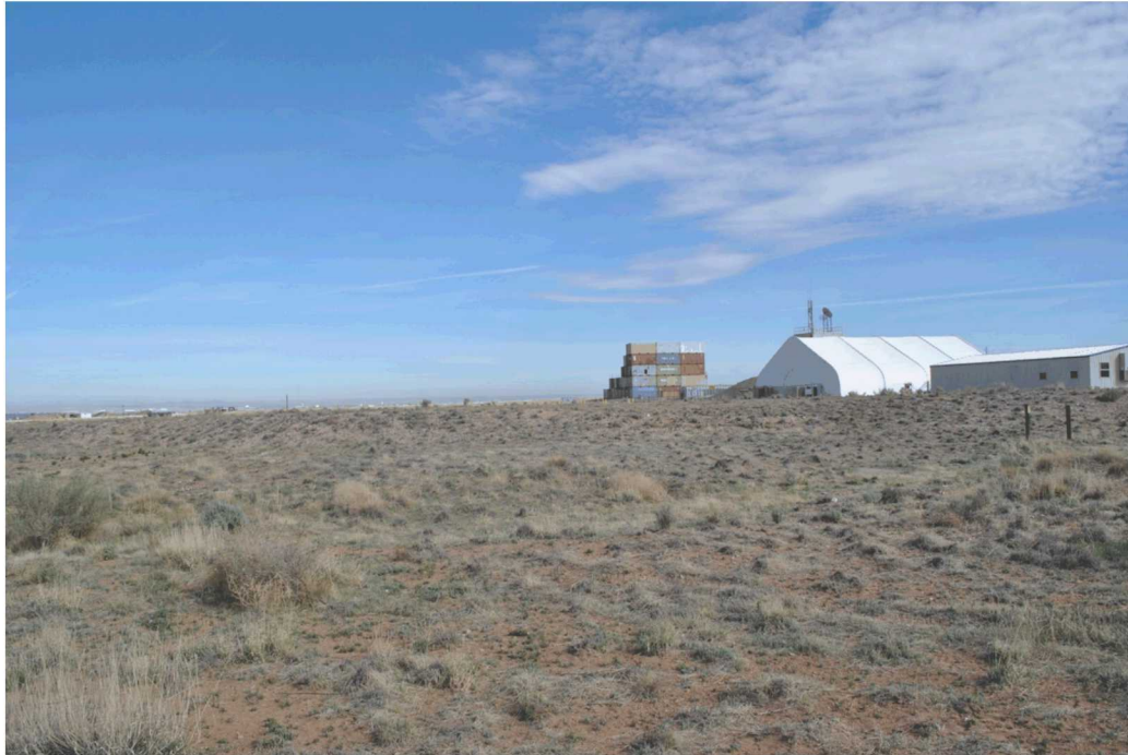
Photo C-2. View from South Looking North
