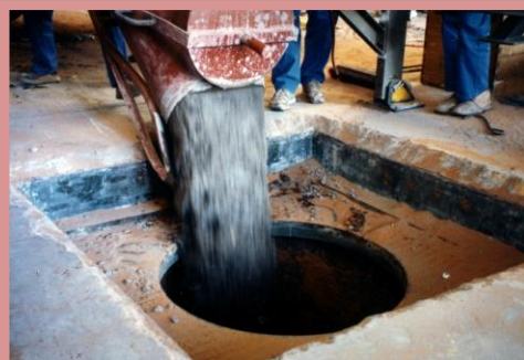
Figure 47. "Rendering harmless" the Kalahari test shafts in South Africa
