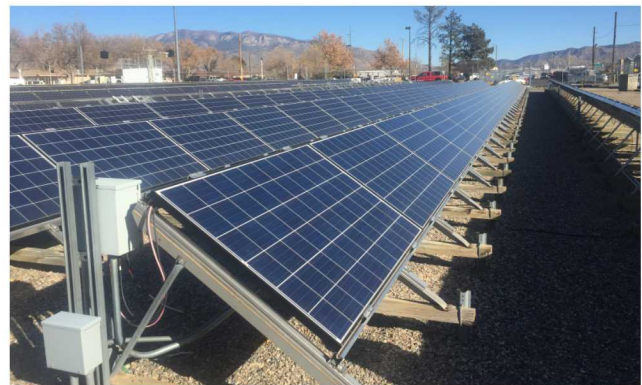
Fig. 1. The solar photovoltaic array was located in Albuquerque, New Mexico. It included two inverters that each supported four strings. The eight strings were routed to a Pordis I-V curve tracing system prior to the combiner box. The combined strings were monitored using the inverters data acquisition system.
