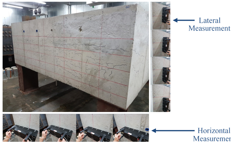
FIGURE 7. Lateral surface grid with lateral MIRA measurements on line A and horizontal MIRA measurements on line 1.
