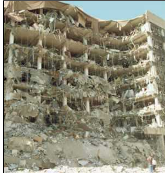
Pre-emptive Reinforcement of Buildings
