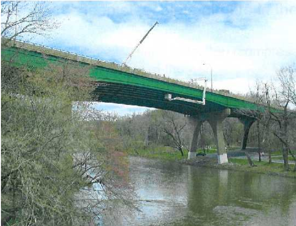
Brandywine River Bridge Interstate Highway 95 Delaware
