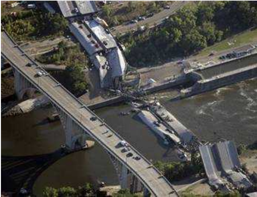
Monitor and Reinforce Bridges
