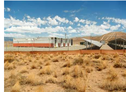
PNM 500 KW solar plant with 250 kW/ 1 MWh Energy Storage
