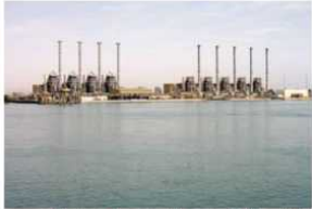
Azzizia desalination plant, Saudi Arabia - Flickr CC BY-NC-SA 2.0 by Waleed Alzuhair
