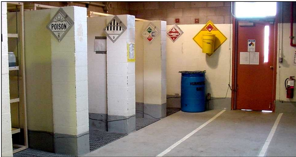
Waste storage bays in Building 959
