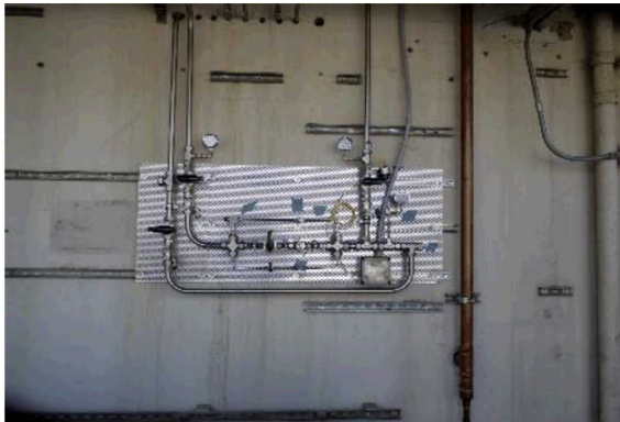
Pressure system design, assemble, test and prepare supporting documentation
