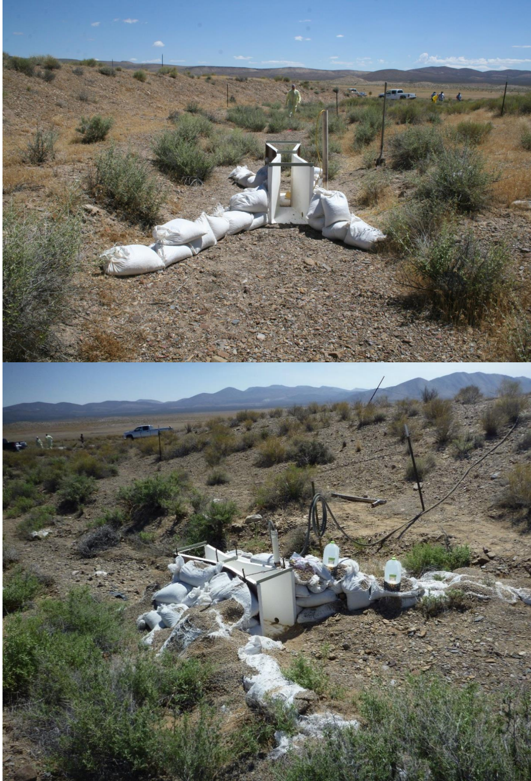
Figure 4. A Parshall flume was installed to measure runoff from the southern portion of the Smoky Site CA. The initial installation (top) was reinstalled and reinforced (bottom) after the flume was washed out in July 2013. The conduit laying on the hillside connects the water pressure sensor to the datalogger.
