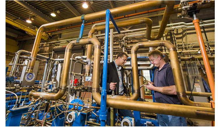
1 MW th -scale sCO 2 Brayton test loop (Source: Sandia National Laboratories)
