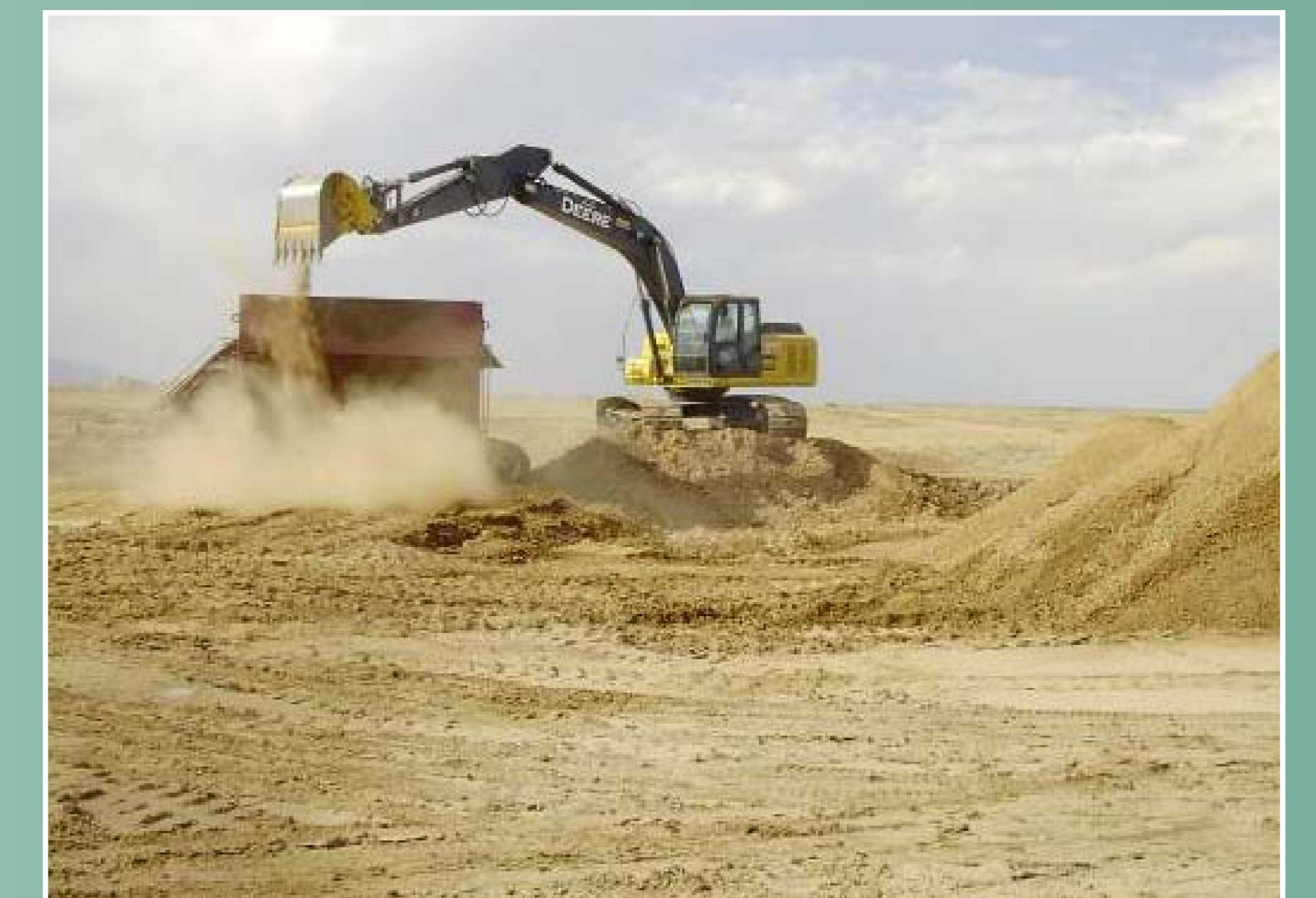
Excavating and screening soils at the SNL/NM Technical Area III borrow pit area in June 2006 to be used for subgrade and ET cover construction.
