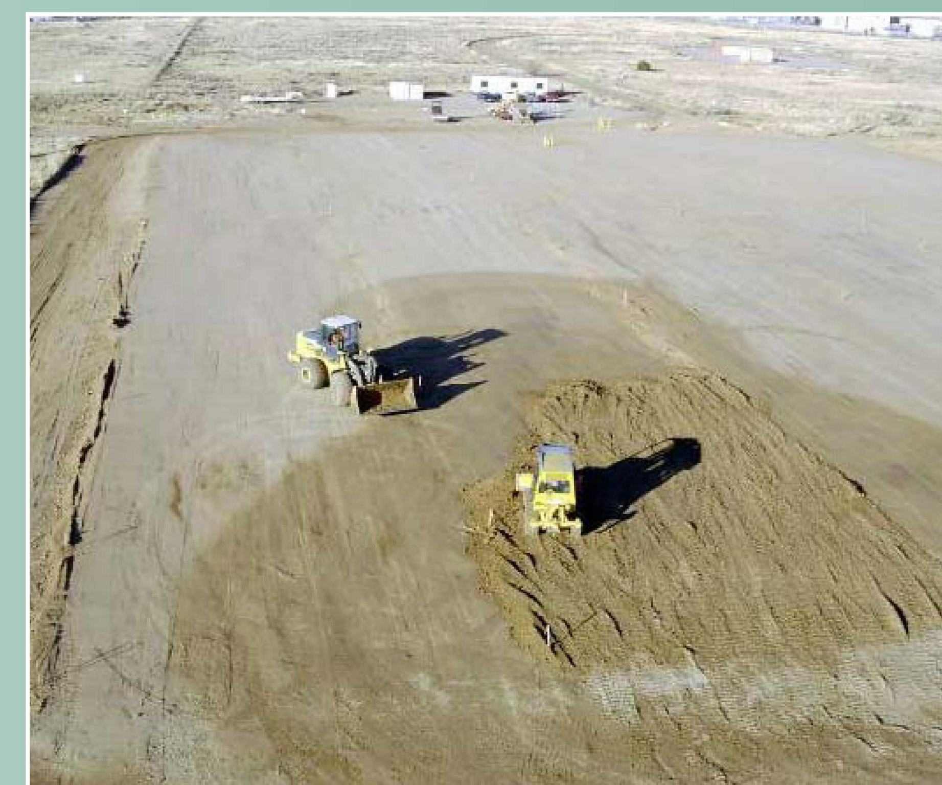
Subgrade preparation in October 2006 – placement and compaction of soil to level the ground surface.
