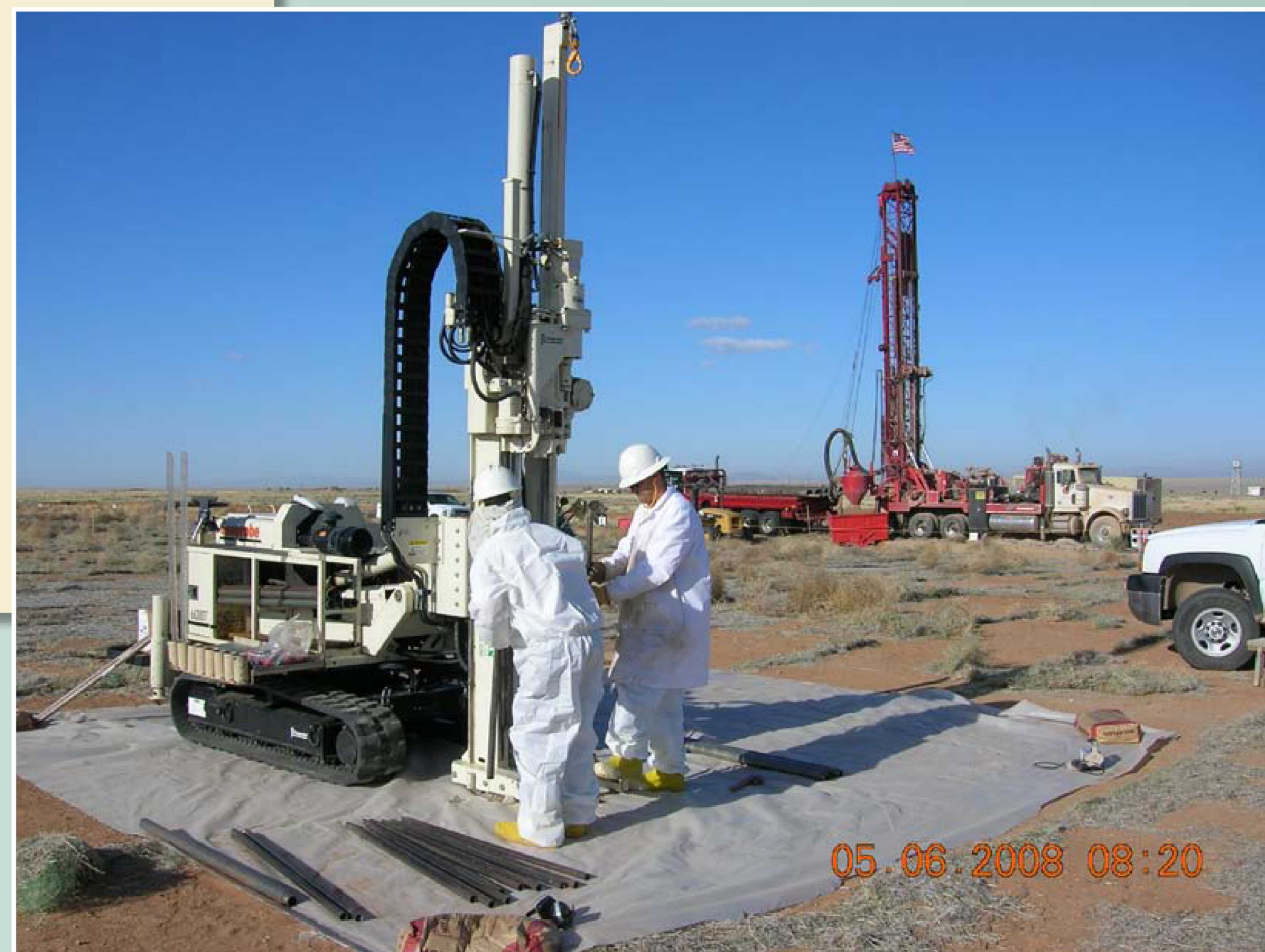
Soil-vapor sampling and new monitoring well drilling (background) in May 2008.
