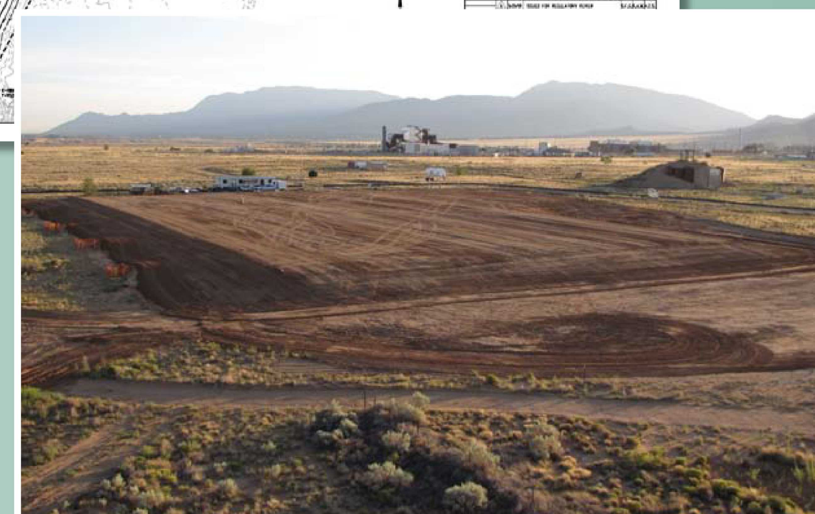
ET cover Topsoil Layer after placement in August 2009.
