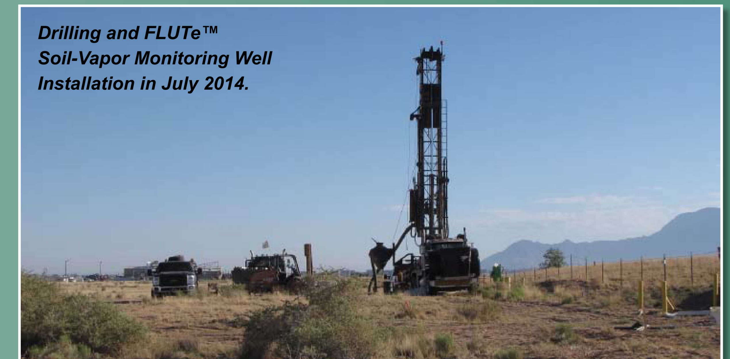
Installation of the FLUTe™ flexible liner for Multi-Port Soil-Vapor Monitoring Well MWL-SV05 in July 2014.
