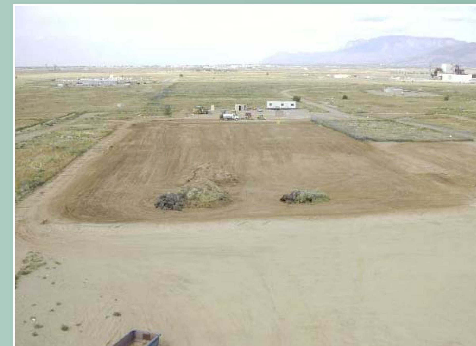
Subgrade preparation field work in October 2006 – removal of existing vegetation prior to leveling the ground surface.
