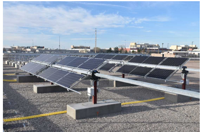
Fig. 4. Single axis tracker for bifacial modules being constructed at Sandia.
