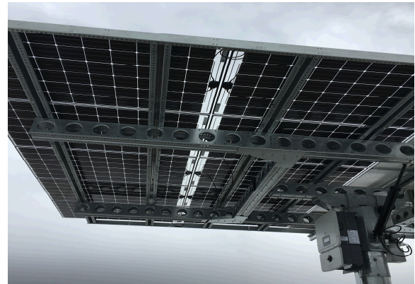
Fig. 13. View of the rear side of the tracker for System 1 showing that support structure blocks the back side of the bifacial modules.
