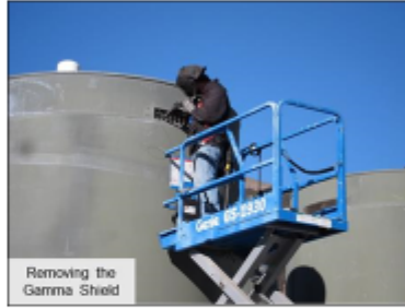
Sampling a HI-STORM 100 canister at the Diablo Canyon ISFSI
