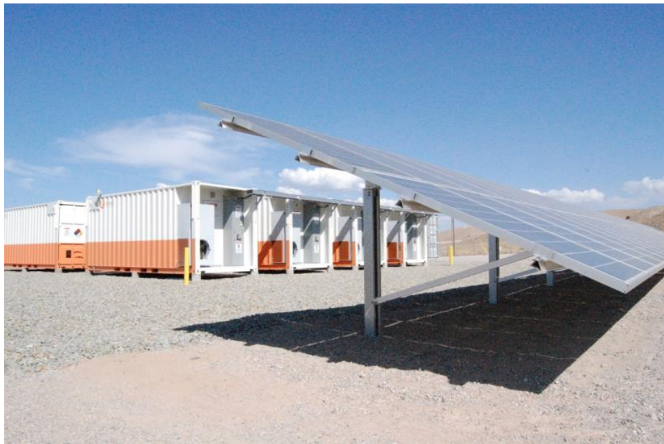
Figure 2: PNM Prosperity project [2].
