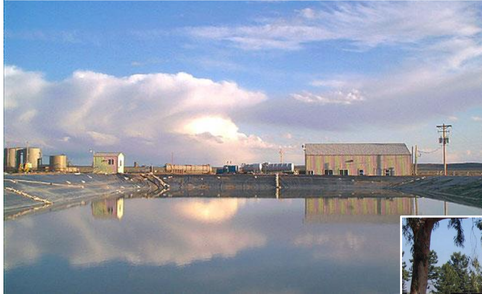
Evaporation pond for produced water
